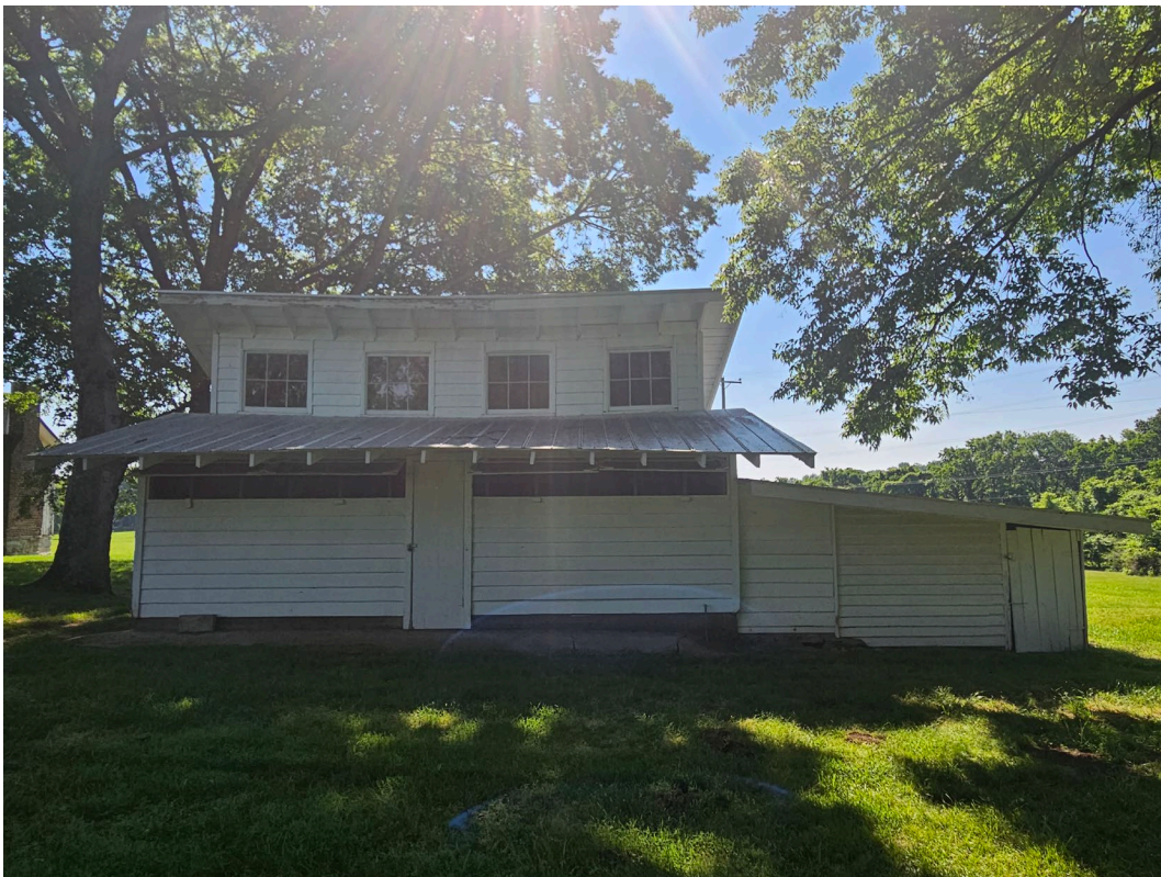
Outbuilding 2; Façade/East elevation.
