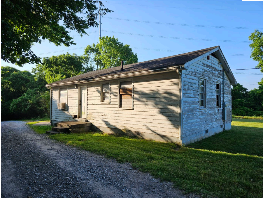
HS-5, 100 Clover Bottom Ave.; Façade/North and East Elevations.
