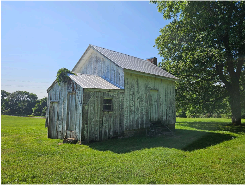
Outbuilding 2; Oblique of Façade/East Elevation and North Elevation.
