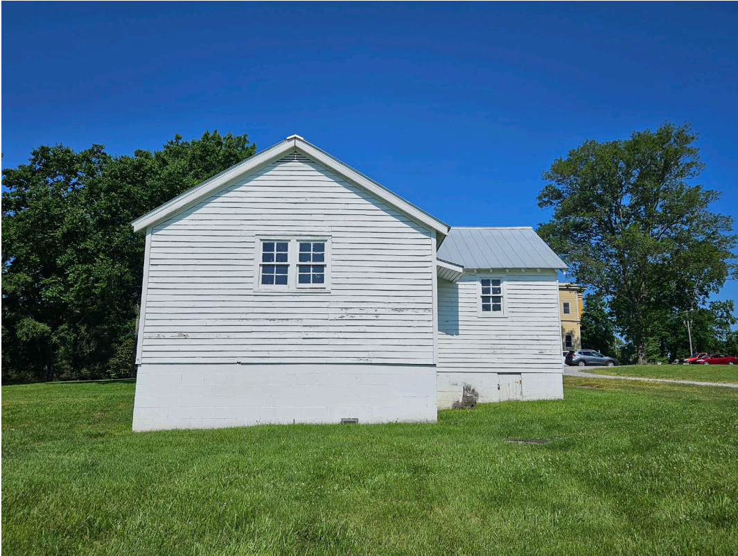
Outbuilding 1; Rear/West Elevation.
