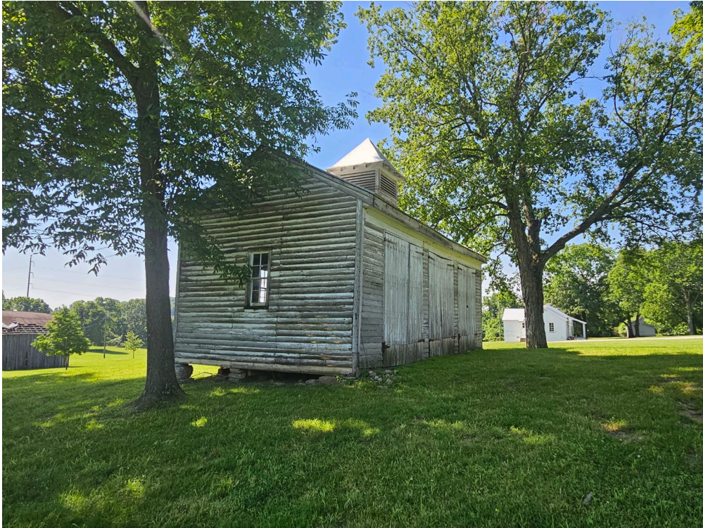
Outbuilding 6; Oblique view of North and East Elevations.
