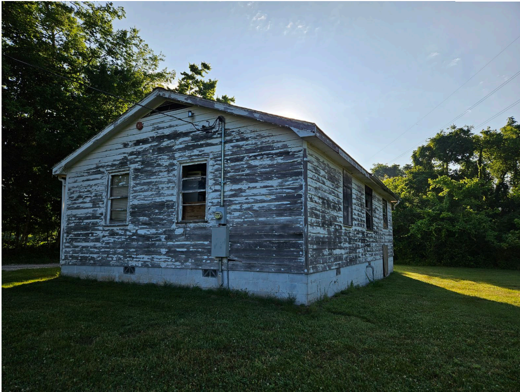
HS-5, 100 Clover Bottom Ave.; East and South Elevations.
