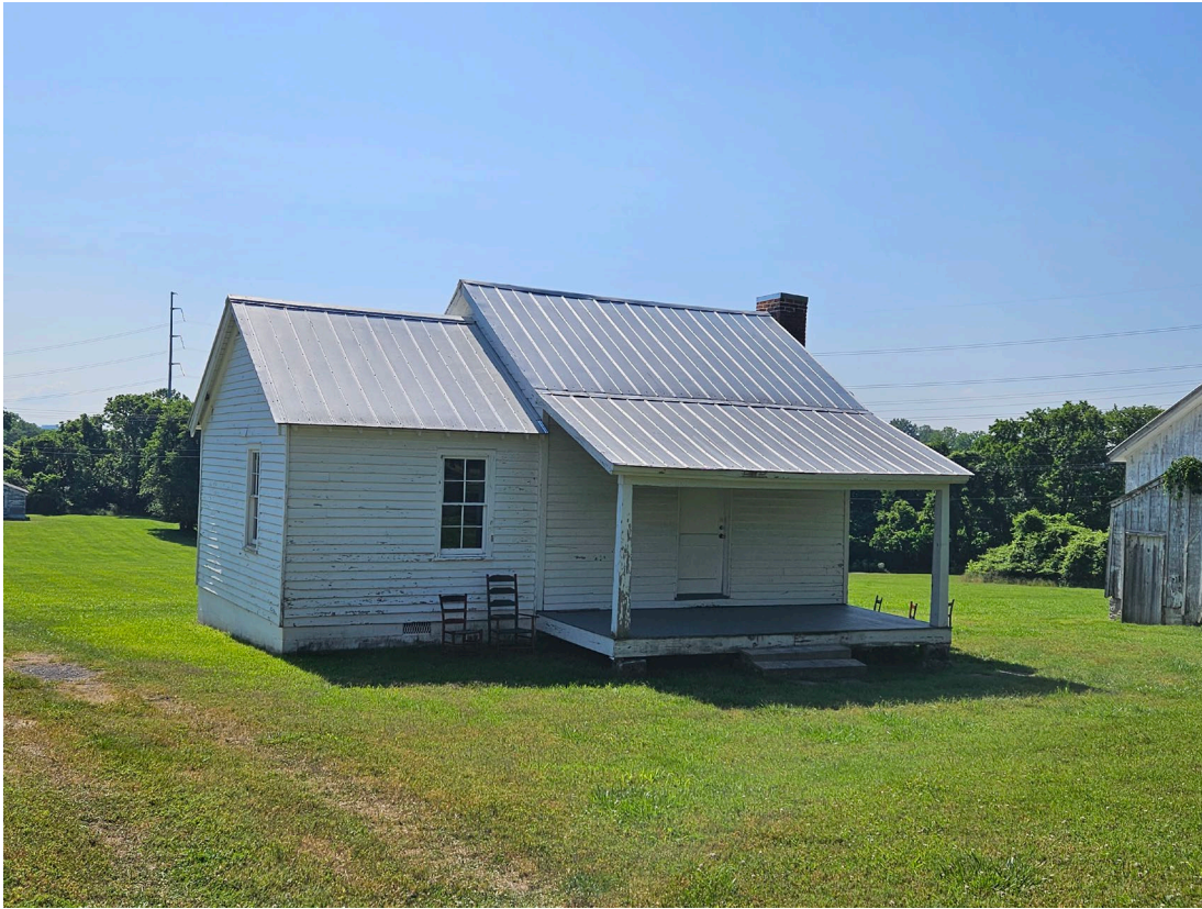
Outbuilding 1; Façade/East Elevation.
