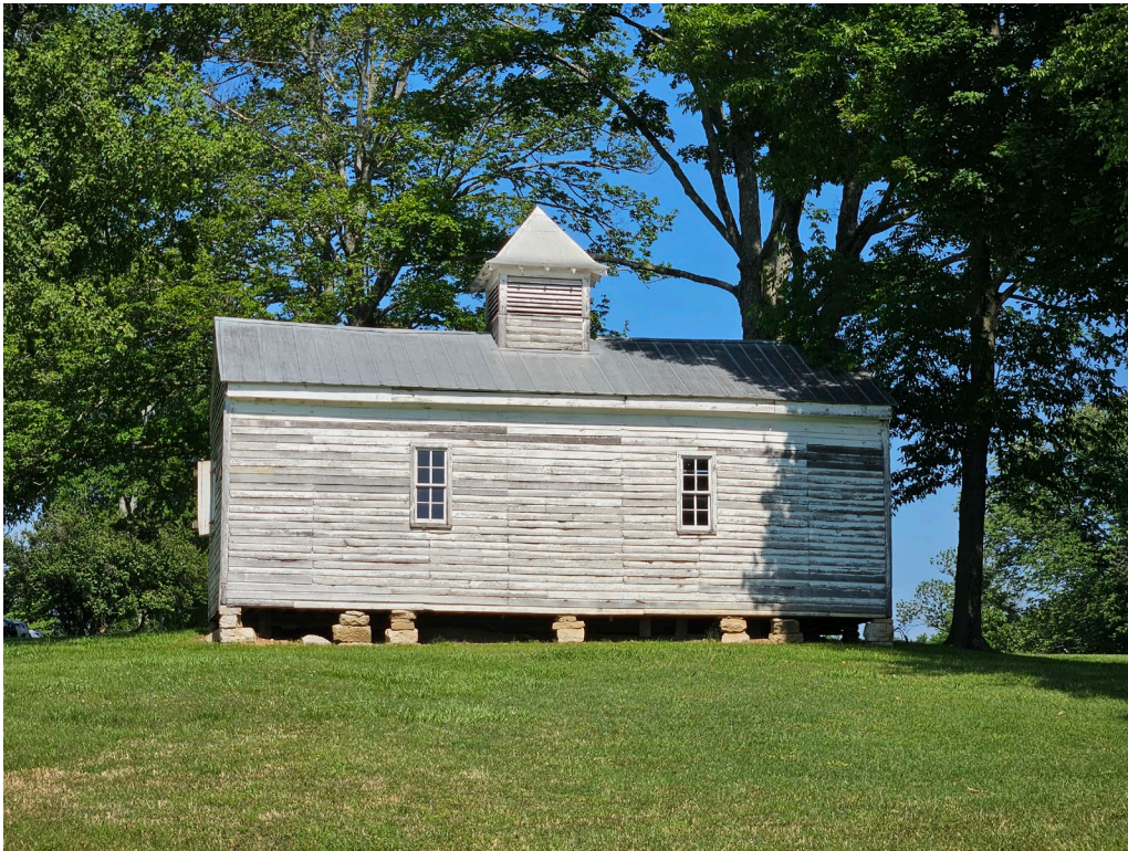
Outbuilding 6; West Elevation.
