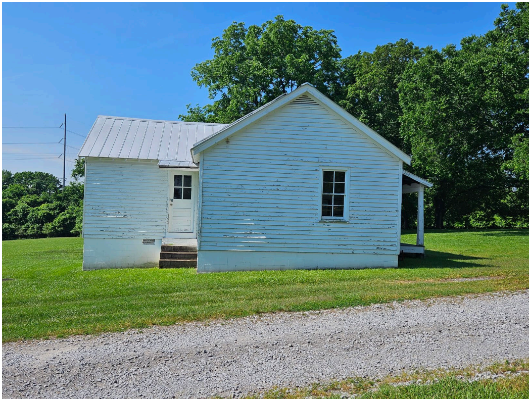
Outbuilding 1; North Elevation.
