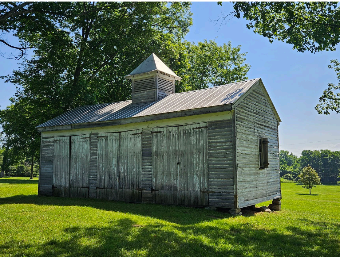
Outbuilding 6; Oblique view of East and South Elevations.
