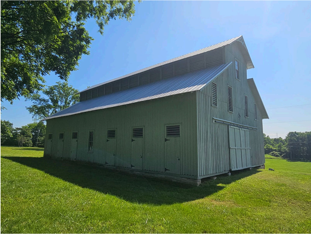
Outbuilding 5; Oblique view of East and South Elevations.
