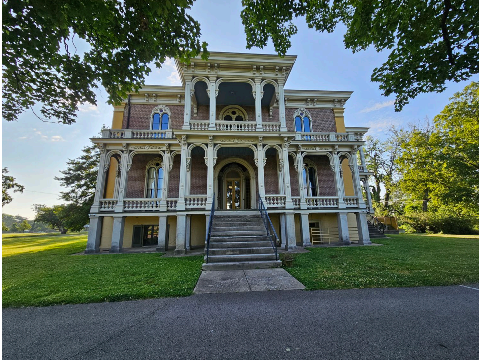
Clover Bottom Mansion; Façade/East Elevation.
