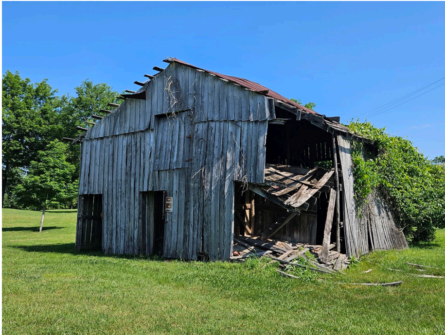
Outbuilding 4; Oblique view of South and West Elevations.
