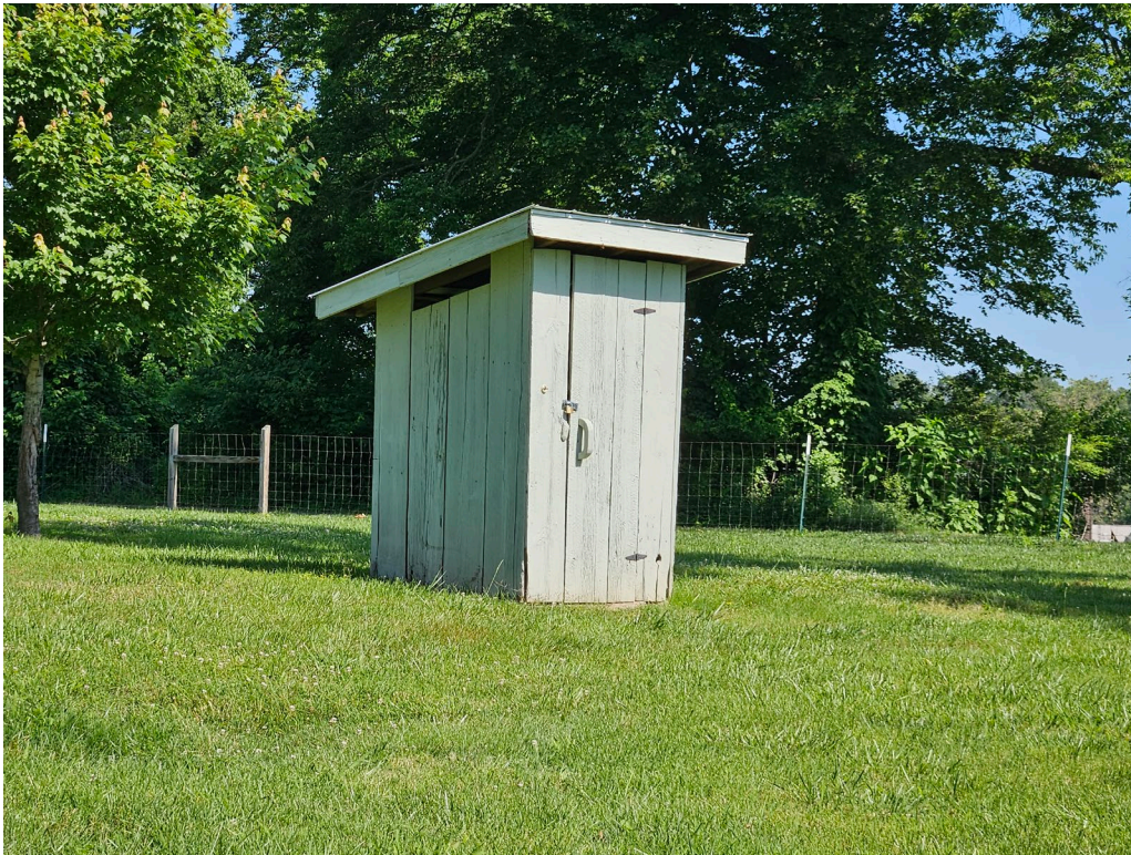
Outbuilding 7; Oblique view of South and West Elevations.
