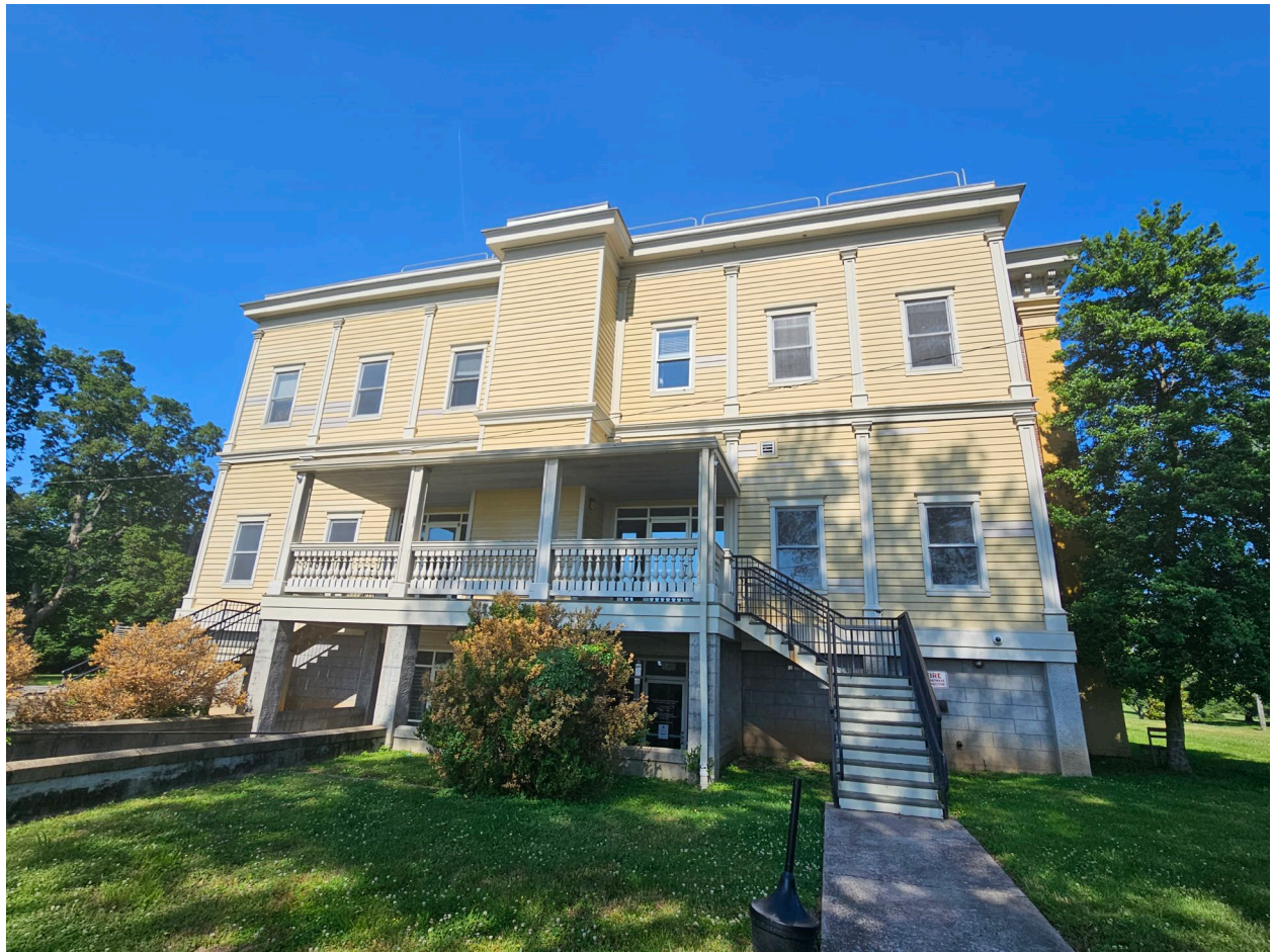
Clover Bottom Mansion; Rear/West Elevation.
