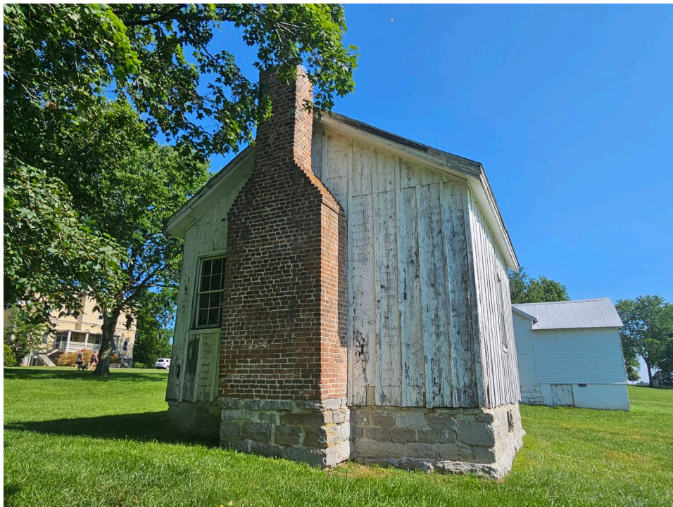
Outbuilding2; South Elevation.
