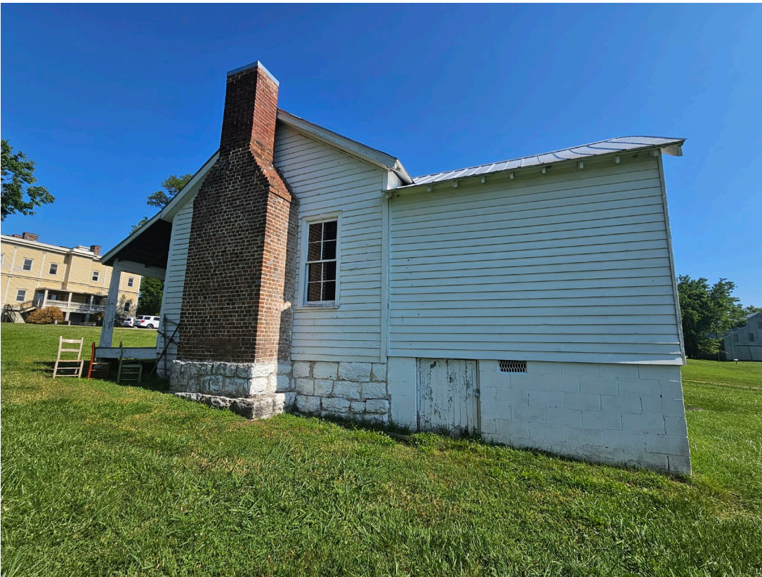
Outbuilding 1; South Elevation.
