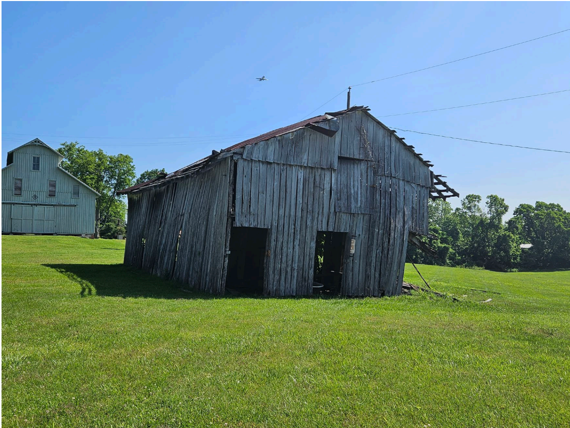
Outbuilding 4; South Elevation.
