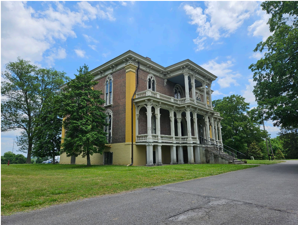
Clover Bottom Mansion; Oblique view of Façade and North Elevation.
