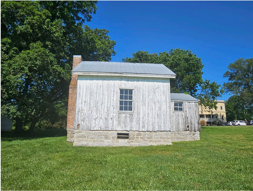
Outbuilding 2; Rear/West Elevation.
