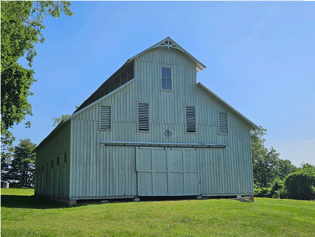
Outbuilding 5; South Elevation.
