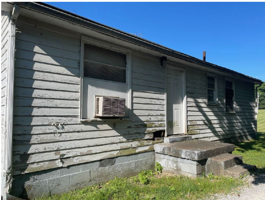
HS-5, 100 Clover Bottom Ave.; Façade/North Elevation.
