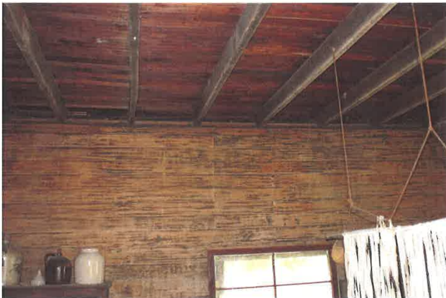
Kitchen - Interior - Roof 1
