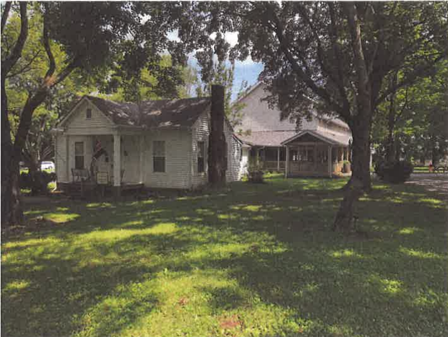
Visitors Center & Offices - Exterior 2
