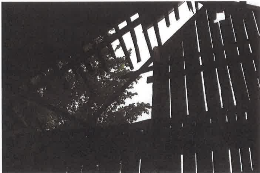
The White Barn Interior - Roof
