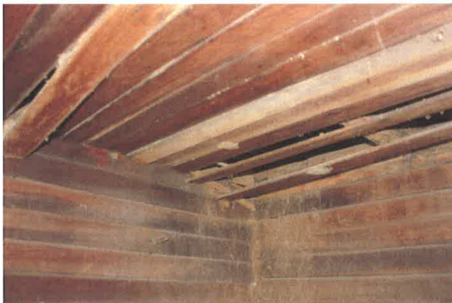
Privy - Interior roof
