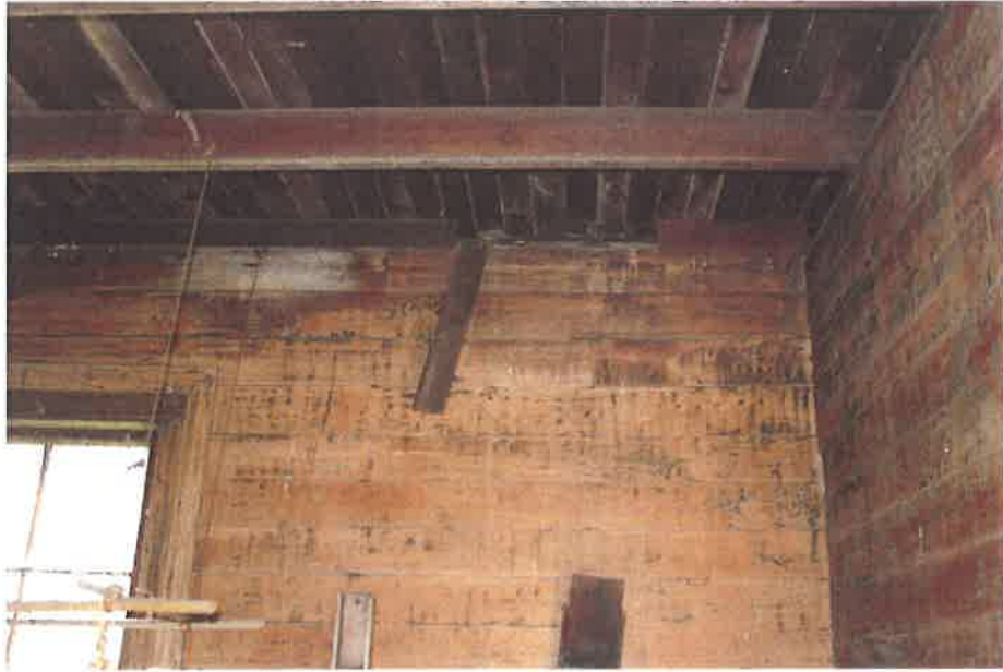
Kitchen - Interior - Roof 2
