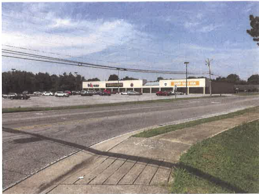
Current View SW Corner - Photo 2 Intersection of Sam Davis Rd. / Nissan Drive
