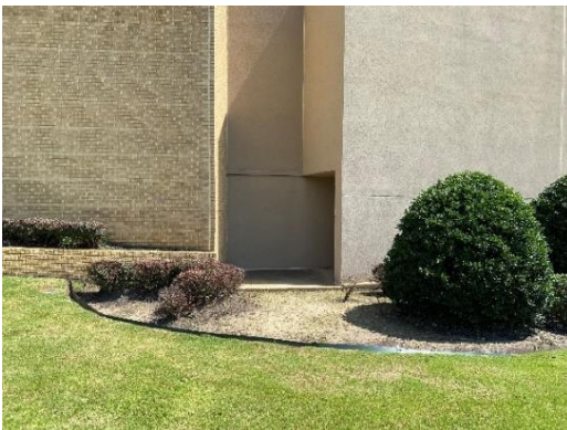
Exit discharge at west exit stair
