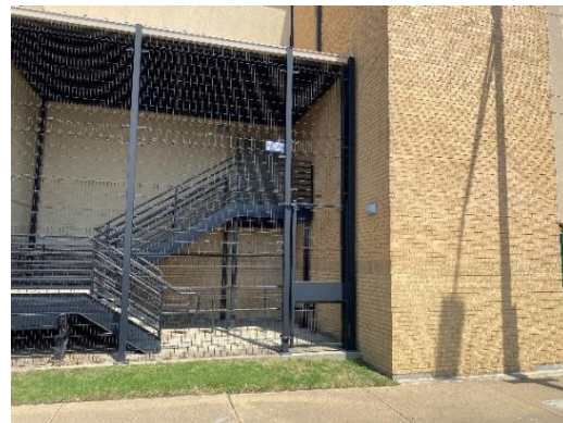
Exit discharge at south exterior stairway
