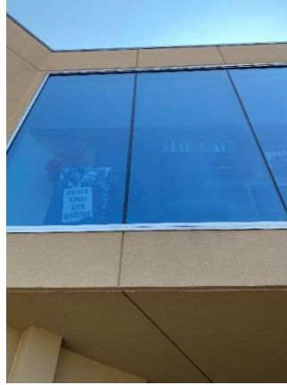
Glazing system needs replacement at gift shop
