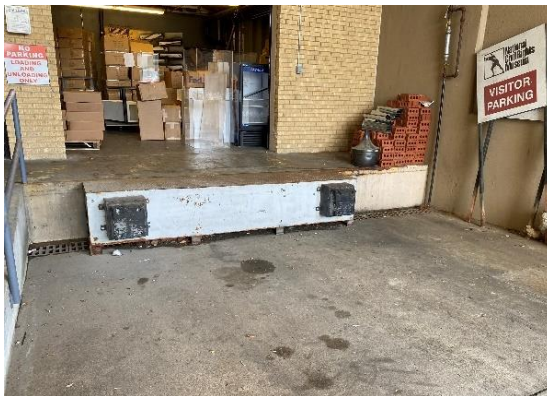
Existing loading dock
