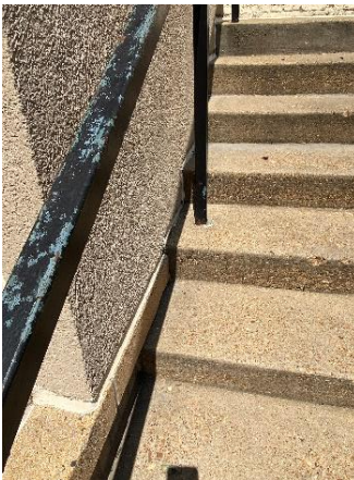
Peeling paint at exterior handrails and guardrails that need refinishing
