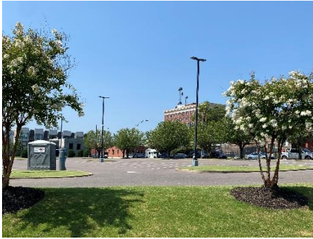
New site lighting at the visitors parking lot
