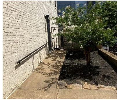
Gate has been secured to mechanical courtyard
