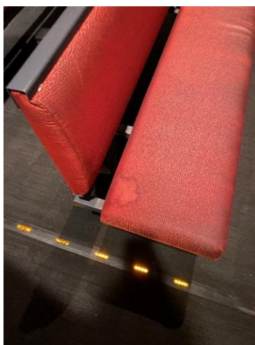
Stained bench upholstery to be replaced in theater spaces
