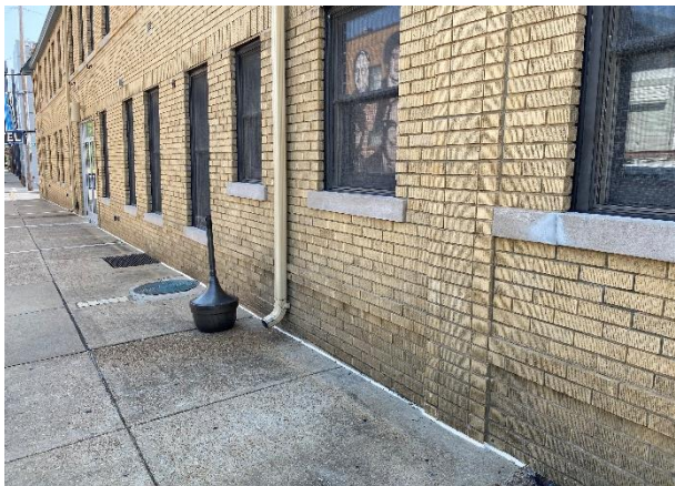
Brick façade around entire perimeter to be cleaned
