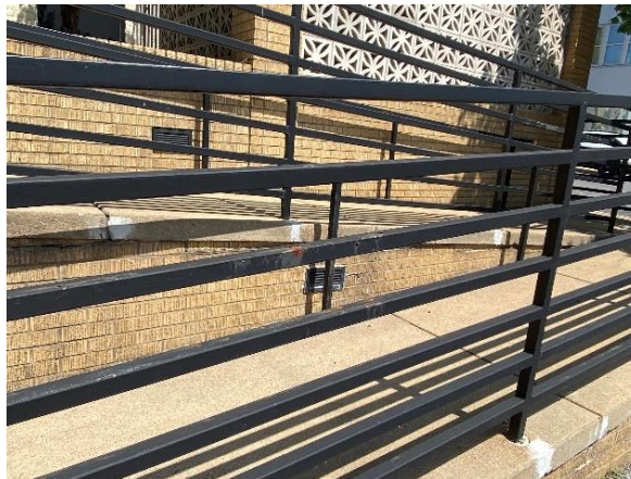
Peeling paint at exterior handrails and guardrails that need refinishing
