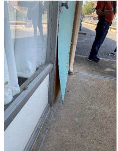
Glazing system needs replacement at gift shop
