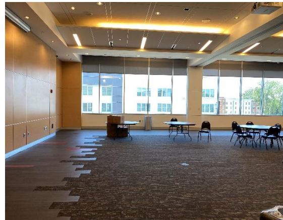
New flooring installed in Hook Hyde Hall
