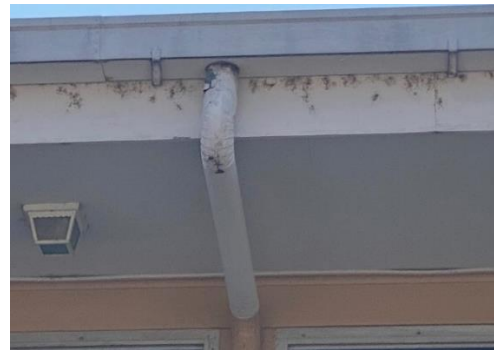
Gutters and downspouts at Lorraine Motel
