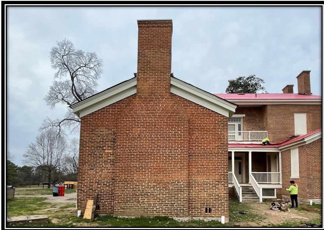
Wood trim repaired and repainted, December 2023.
