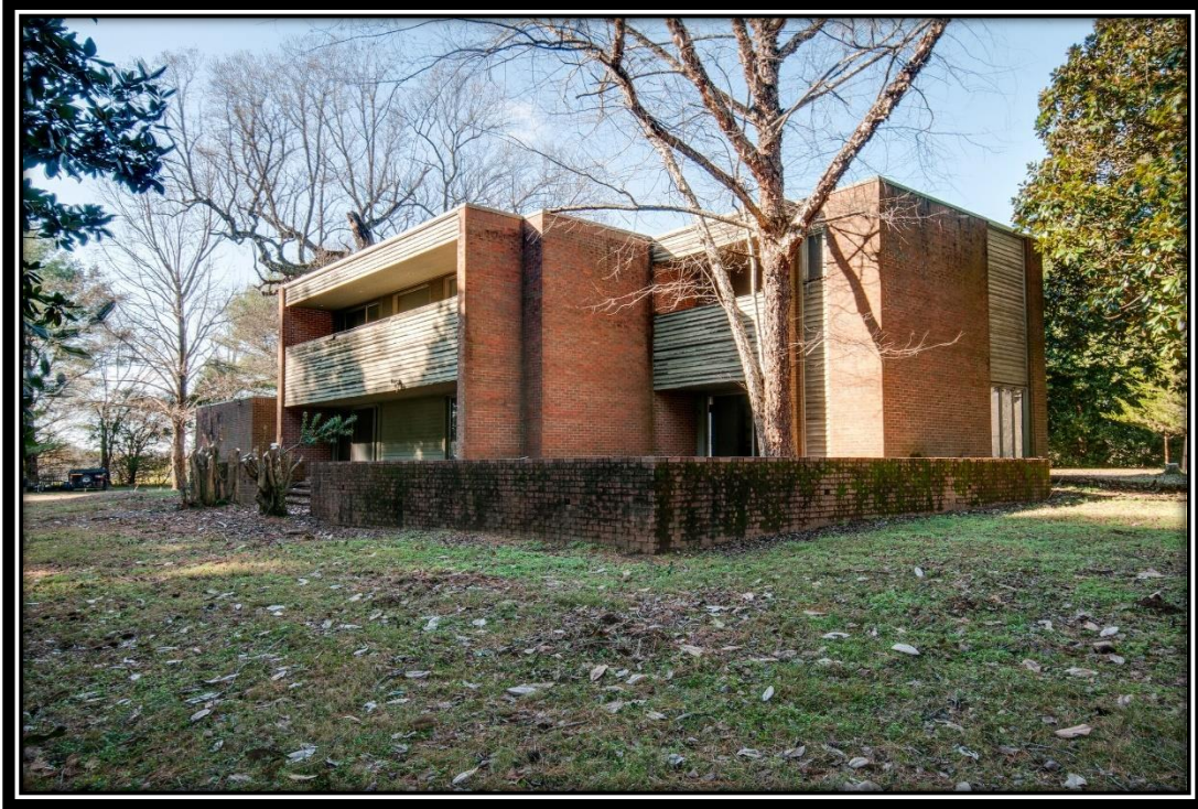
Director's Residence north and east elevation, December 2022.
