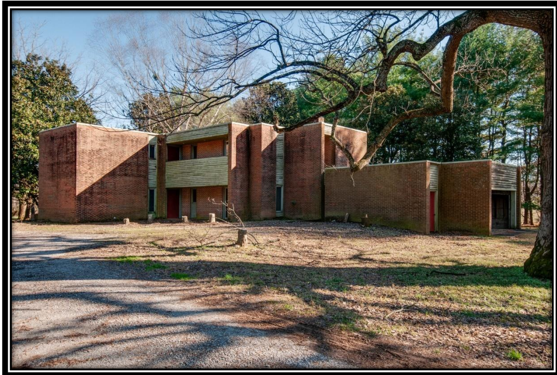
Director's Residence south and west elevations, December 2022.
