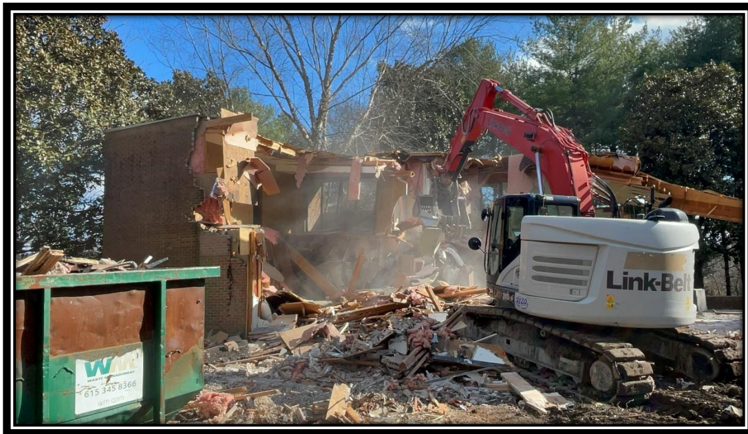
Demolition underway in January 2023.
