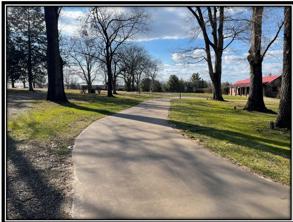
Above, pathway conditions before replacement and below, after.
