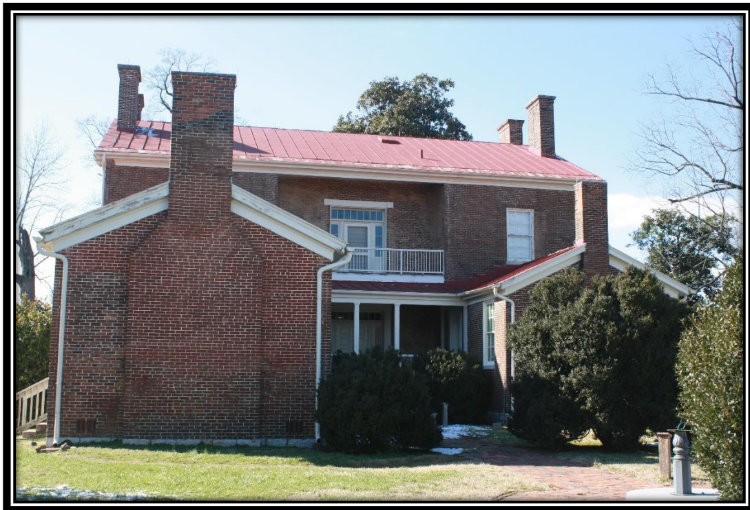
Tulip Grove's c.1964 roof will be replaced in early 2024.
