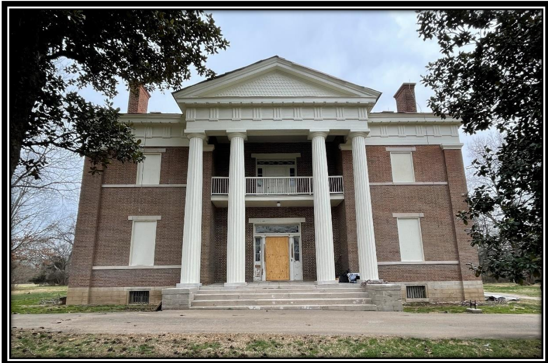
Tulip Grove front façade after wood repairs and repainting.
