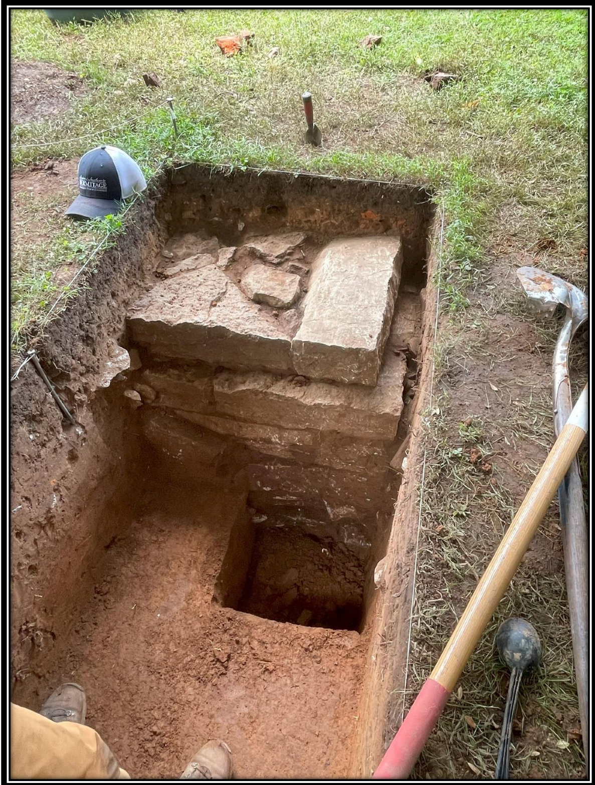
Archaeologists discovered a previously unknown foundation and root cellar within 30 feet of Tulip Grove Mansion. This building may have been a detached kitchen.
