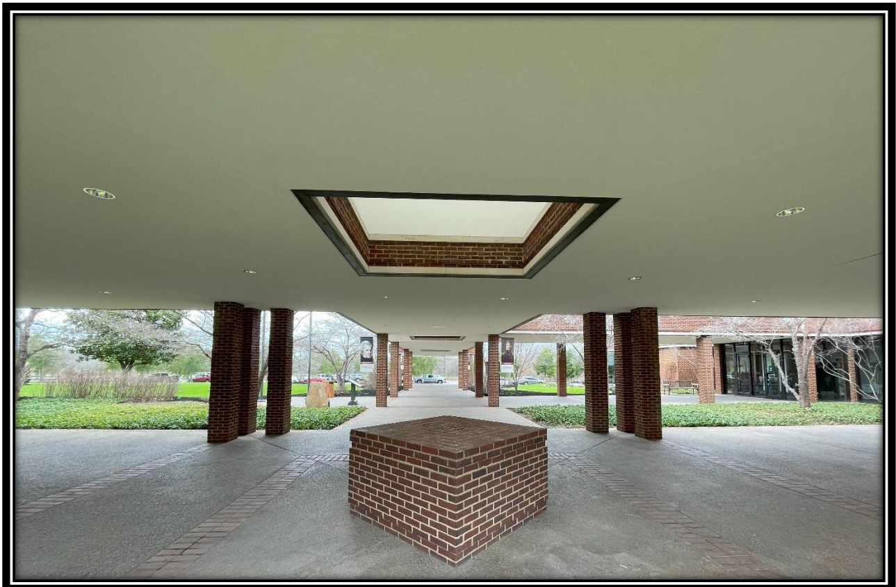
The Visitor Center canopy ceiling after replacement, completed early 2024.
