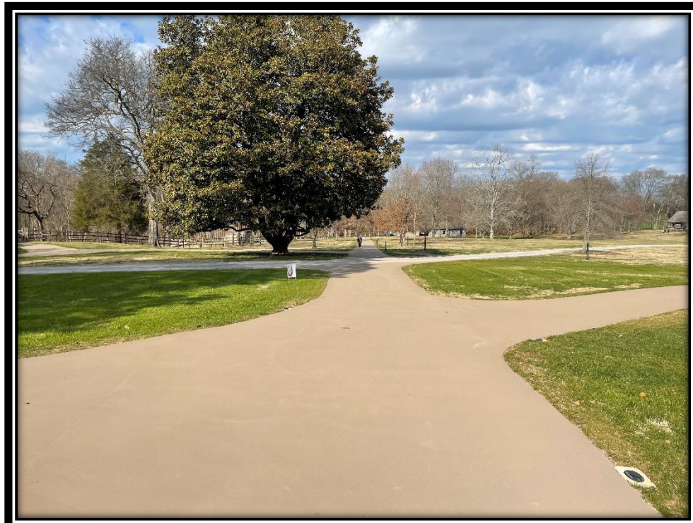
Above, pathway conditions before replacement and below, the new pathway.
