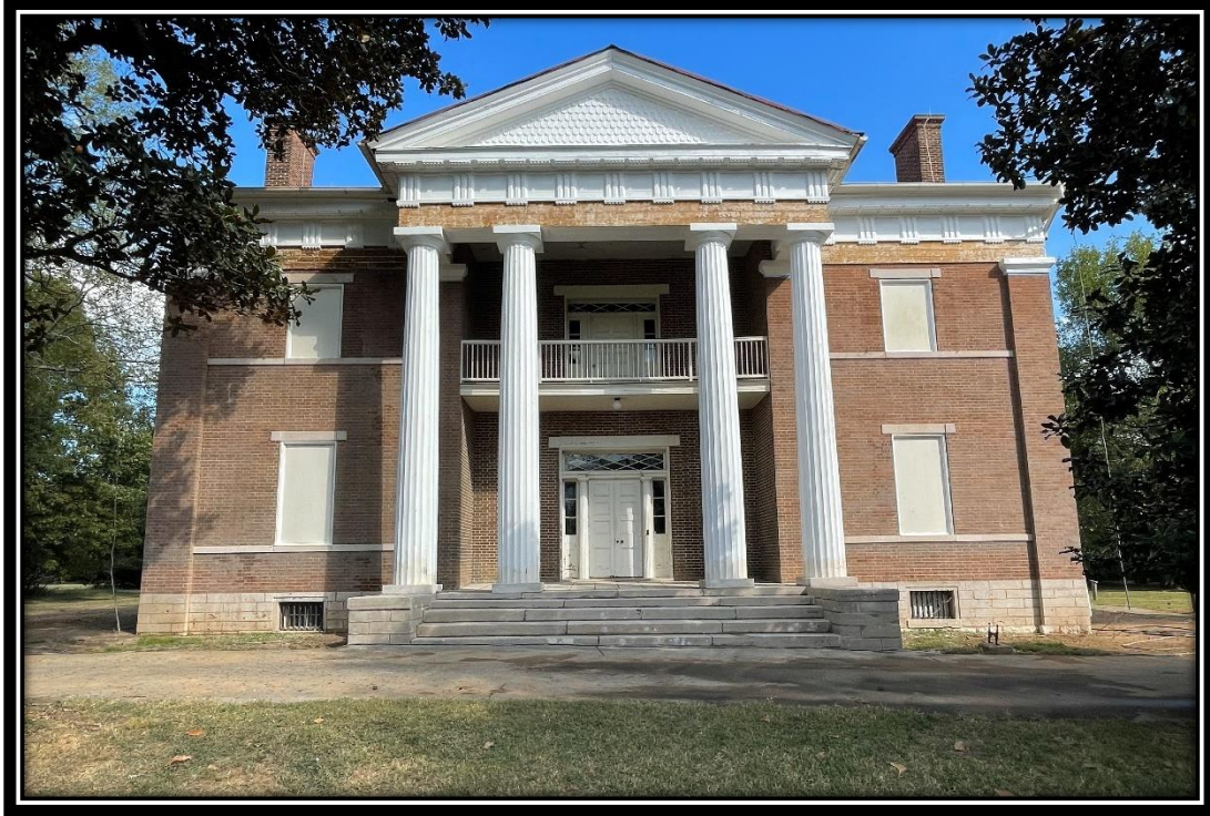
Tulip Grove front façade undergoing repairs and paint prep, September 2023.
