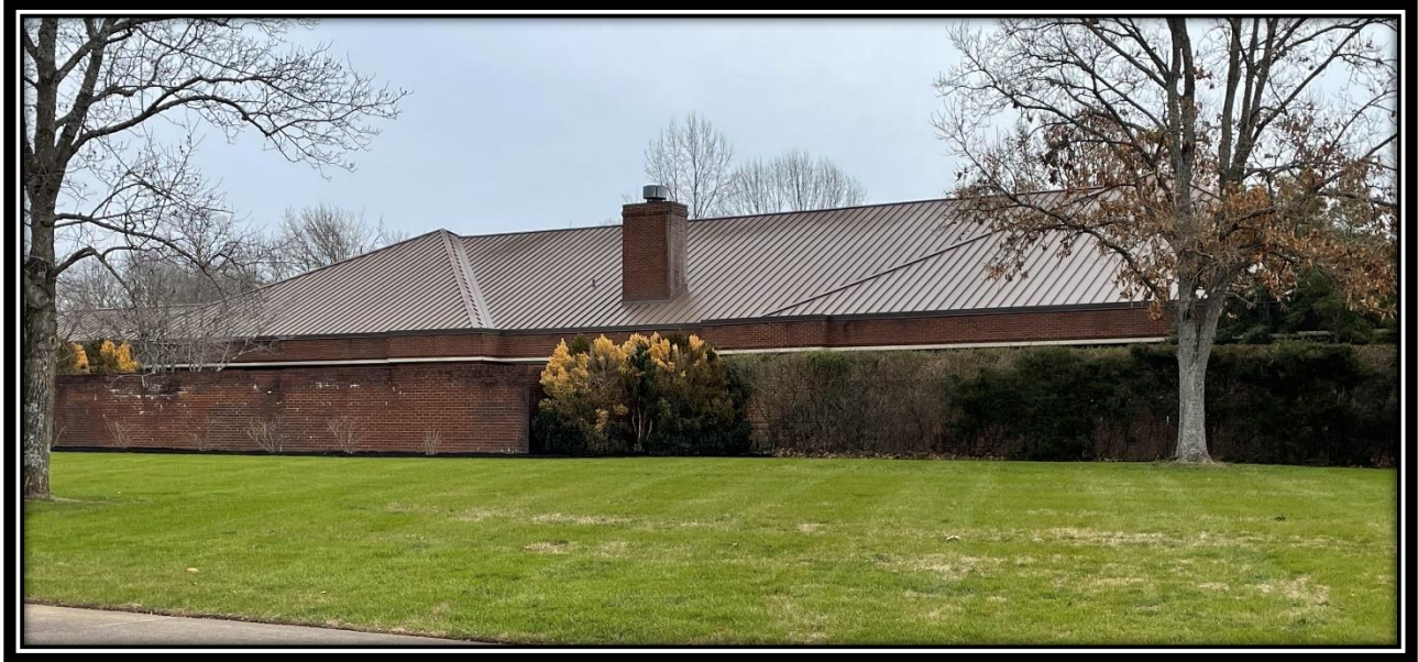
The Andrew Jackson Visitor Center Roof after seal coating, November 2023.
