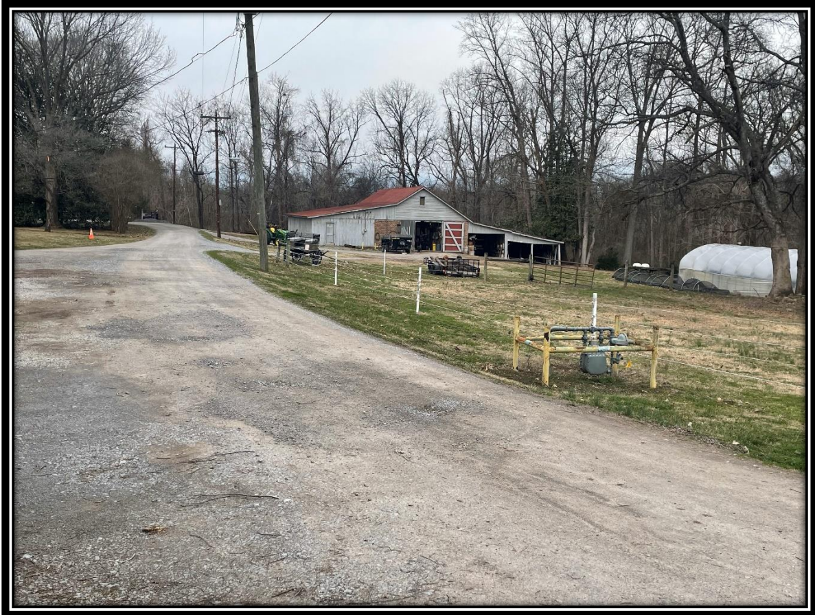
The 1936 Storage Barn and a modern greenhouse are also located in the historic core. A Jackson Era log barn stood where the gas meter stands and the utility poles pass overhead. Converting these site operations areas to public learning spaces would allow the Andrew Jackson Foundation to tell a more complete story of The Hermitage and Andrew Jackson.
