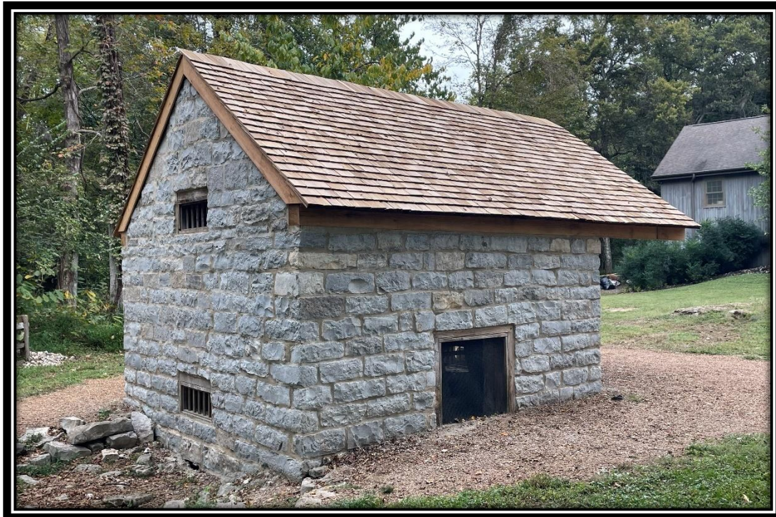
The Hermitage Springhouse pre and post repair, 2021 and 2023.
