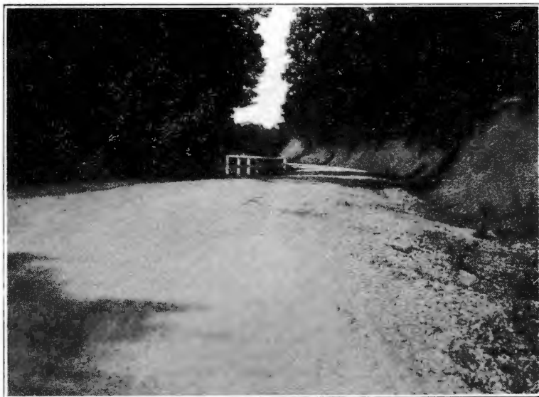
Federal Aid Project No. 6—Washington County. Bituminous Macadam.
