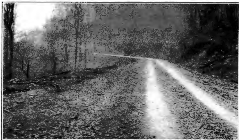
Road over famous Montecle Mountain being built with State Highway Department forces. The stone surfacing was completed on this section December 20, 1924.
