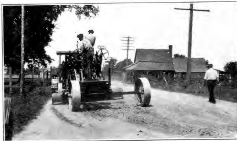
Showing Operation of Reshaping Old Macadam Road by State Maintenance Outfit.
