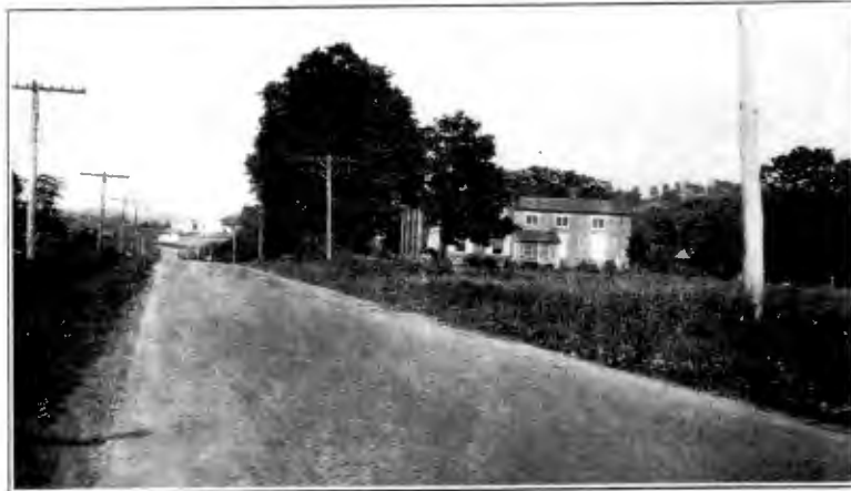
Federal Aid Project No. 41—Knox County. Kentucky Rock Asphalt Surface.
