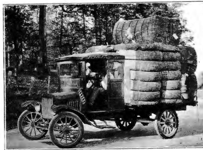
Overloaded Truck—A Menace to Roads.
