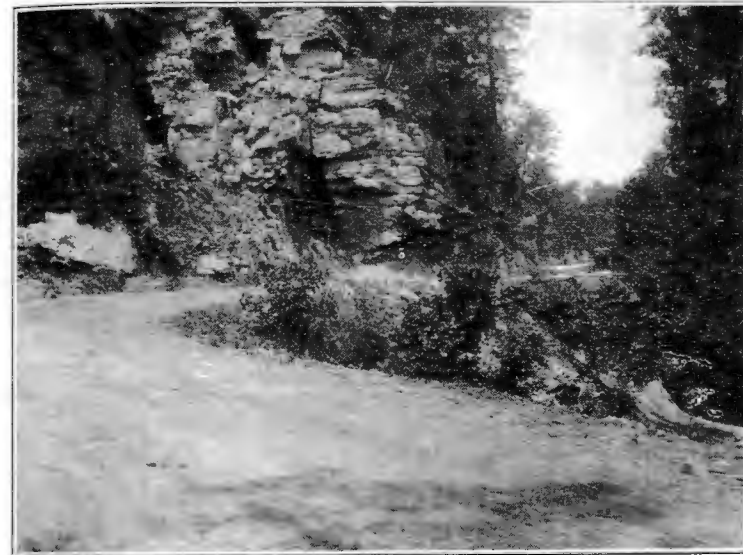
Federal Aid Project No. 24—Marion County. Bituminous Macadam.
