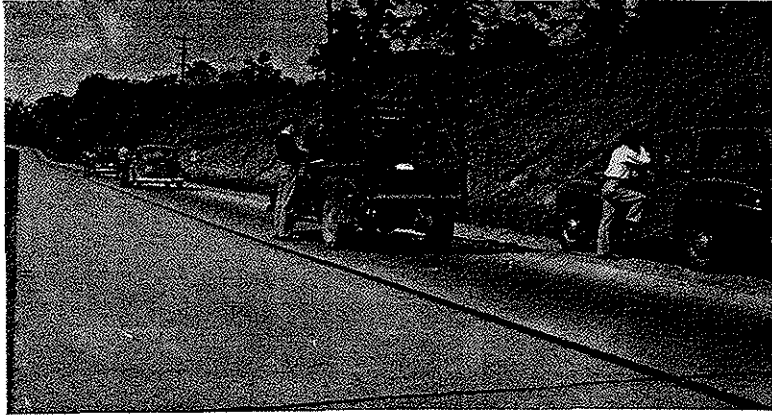
Origin and Destination studies are made to determine the travel desire of motorists in order to better plan for facilities to satisfy this desire.
