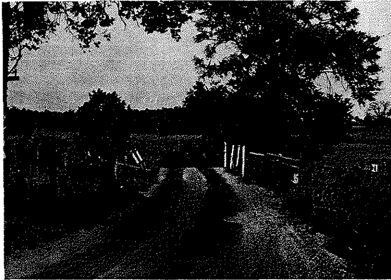
These two photographs show typical conditions on the Rural Roads System which should be improved. The road in Carroll County carries 150 vehicles per day, is narrow and crooked, lacks proper drainage and needs an improved surface. Nearly 500 vehicles per day cross the bridge in Wilson County. The condition of guard rails shows the bridge is too narrow for safe driving. During storms water overflows both approaches.
