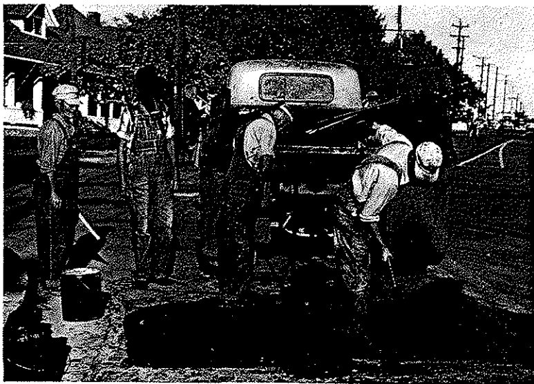
These pictures show the Maintenance Department patching and resurfacing with bituminous material. These are only two phases of the operation of this many-faceted organization.
