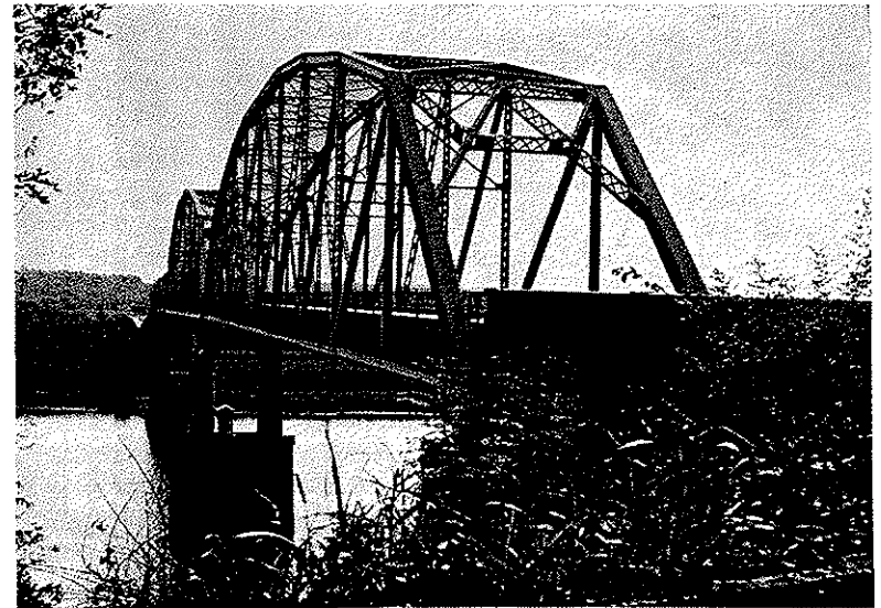
Spanning the Tennessee River, the Alvin York Bridge, in the picture, represents the toll bridges built to facilitate the crossing of the major rivers in Tennessee.
