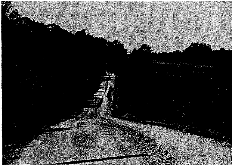
These two photographs show typical conditions on the Rural Roads System which should be improved. The road in Carroll County carries 150 vehicles per day, is narrow and crooked, lacks proper drainage and needs an improved surface. Nearly 500 vehicles per day cross the bridge in Wilson County. The condition of guard rails shows the bridge is too narrow for safe driving. During storms water overflows both approaches.
