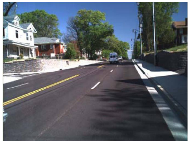
A cross-section with reduced lane widths in Jackson, TN reflects TDOT's flexibility.
