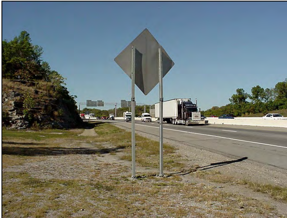
Photo 4: Existing Rock Material Between Exit Loop Ramp and Entrance Ramp
