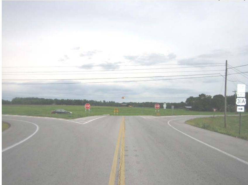
View is westbound at the US 31A (SR 11) intersection.
