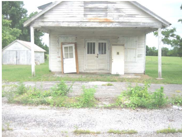
View of potential abandoned UST's
