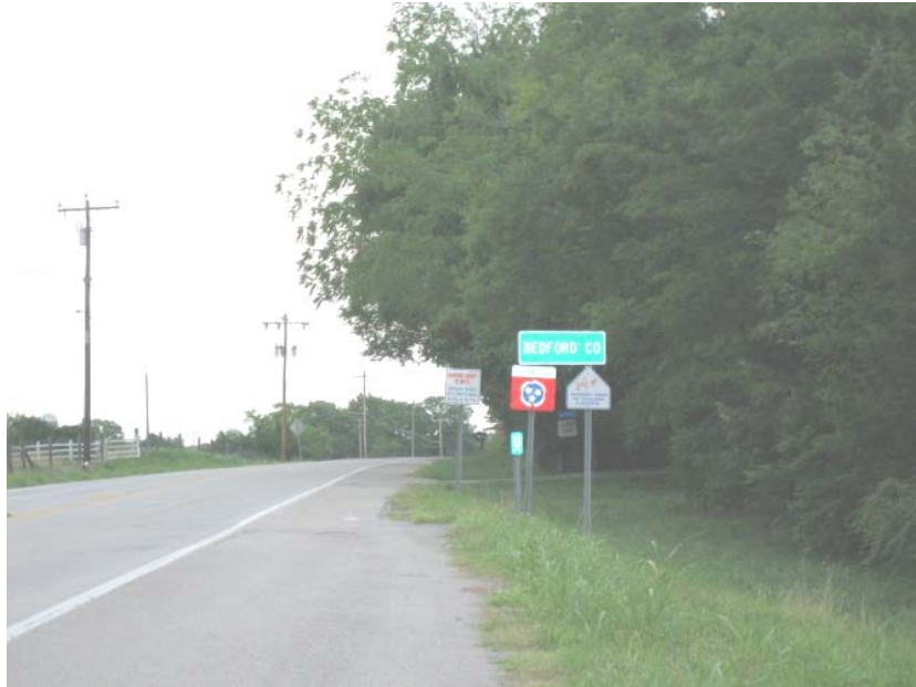
View of shoulder transition at county line
