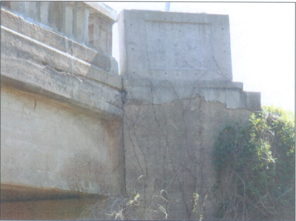
RECASTED WINGWALL ON RIGHT UPSTREAM SIDE OF EXISTING BRIDGE
