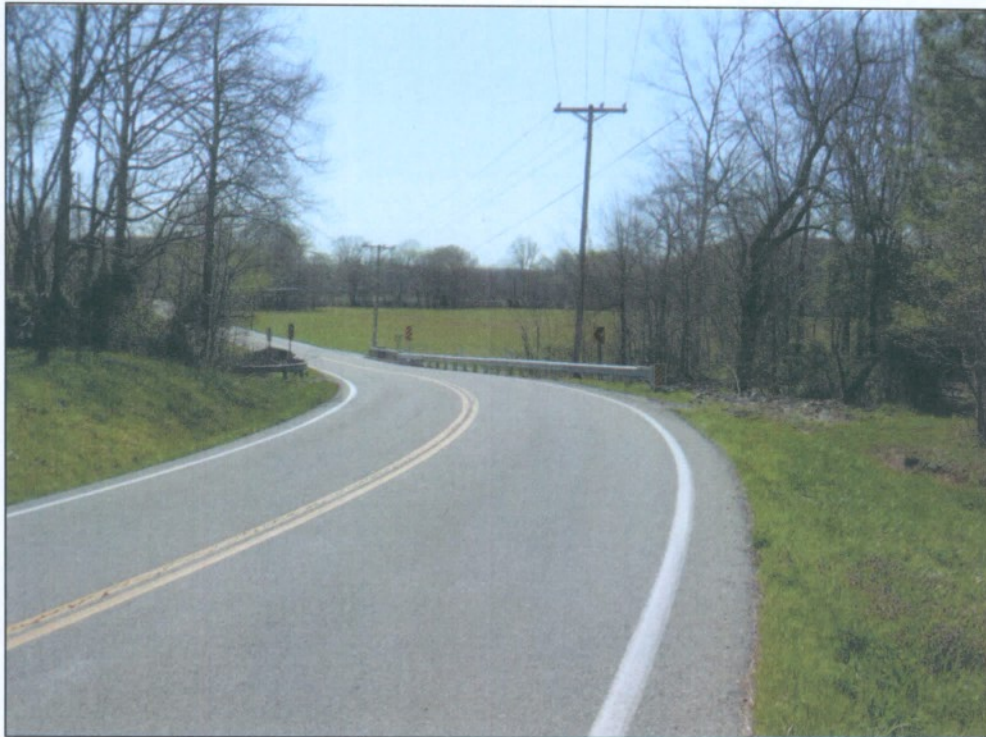
STATE ROUTE 46 EASTBOUND APPROACH TO BRIDGE
