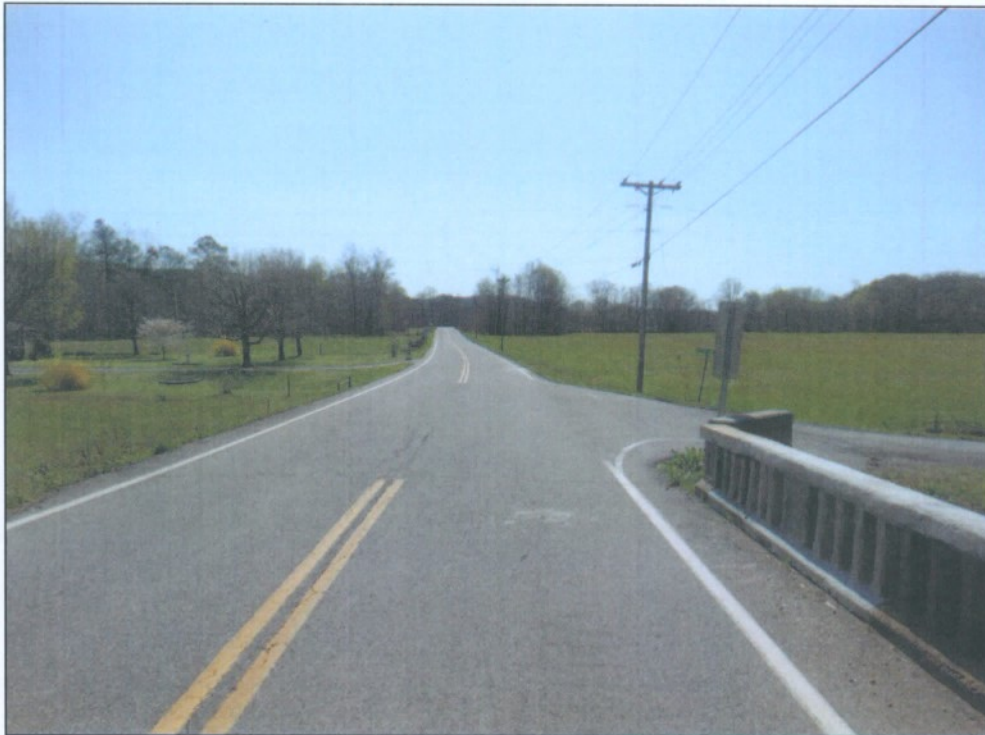
STATE ROUTE 46 EASTBOUND APPROACH FROM BRIDGE
