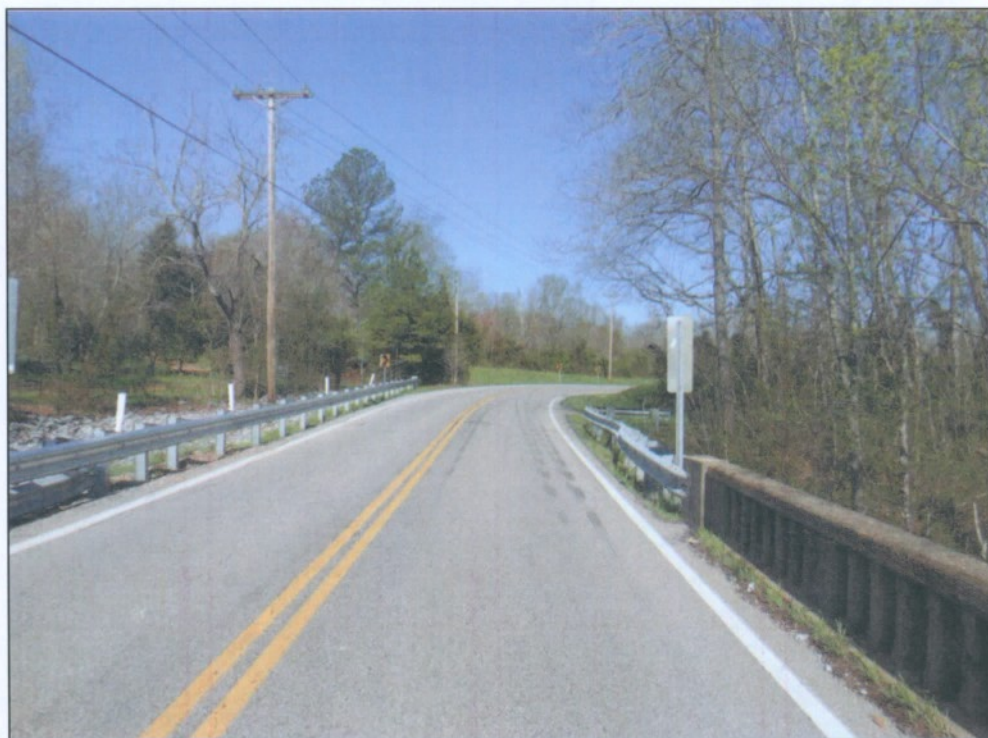
STATE ROUTE 46 WESTBOUND APPROACH FROM BRIDGE
