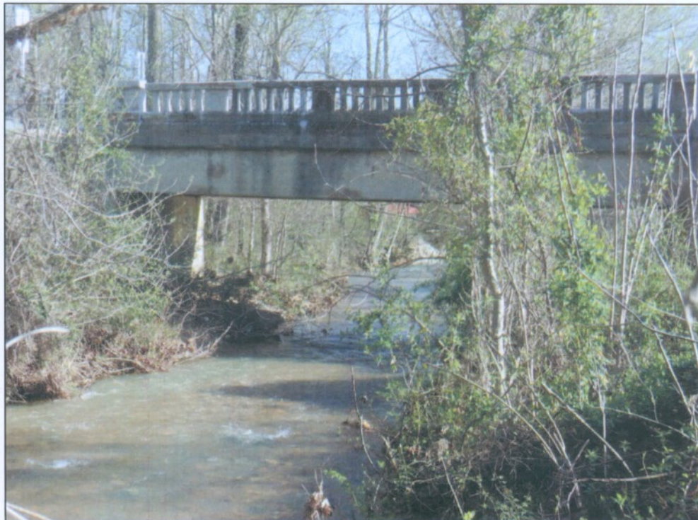
BRIDGE INLET (SOUTH SIDE OF STATE ROUTE 46)
