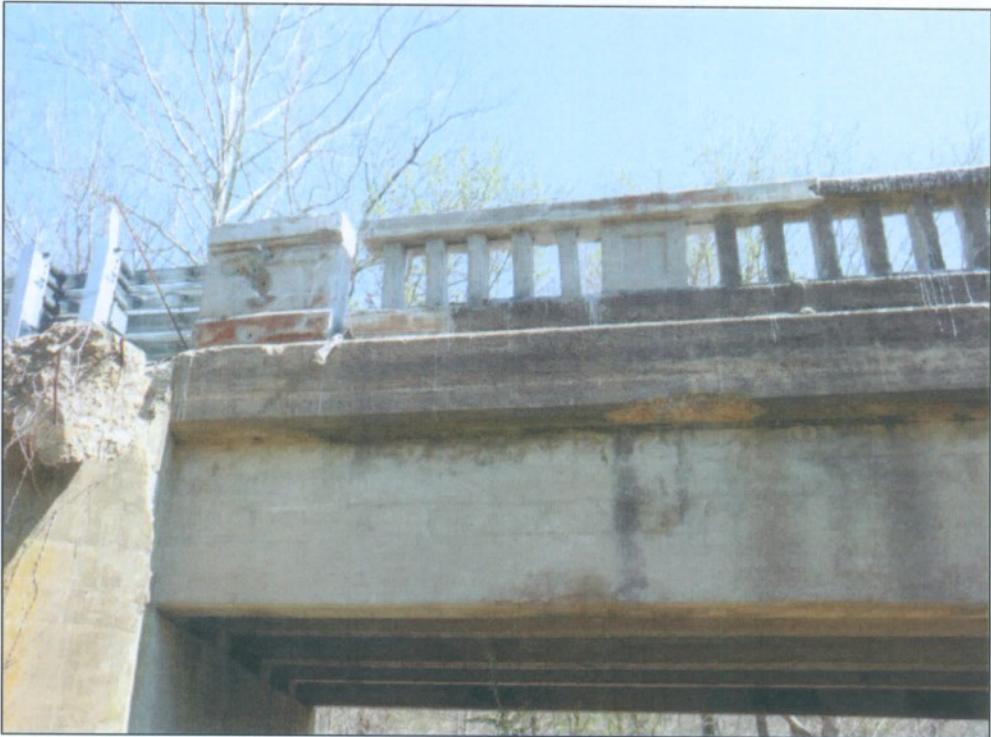
REPLACED BRIDGE RAIL ON UPSTREAM SIDE OF EXISTING BRIDGE
