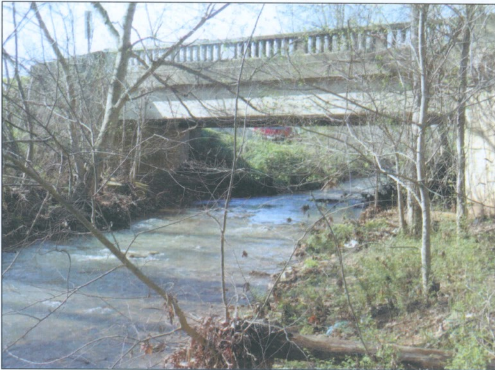
BRIDGE OUTLET (NORTH SIDE OF STATE ROUTE 46)
