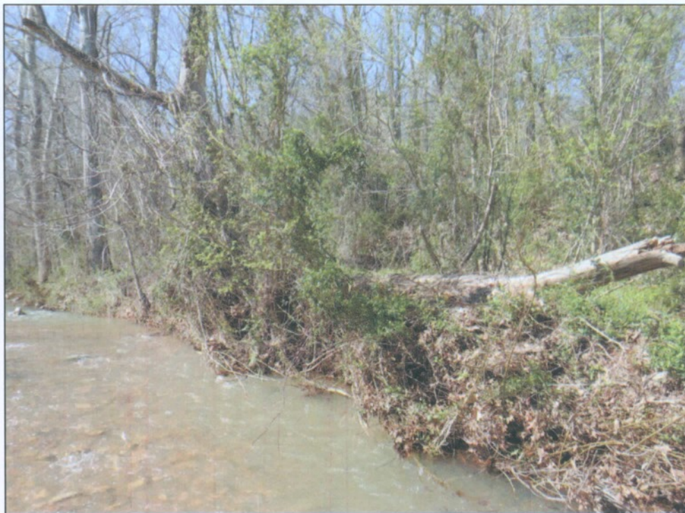
BRANCH LEFT UPSTREAM OF THE EXISTING BRIDGE
