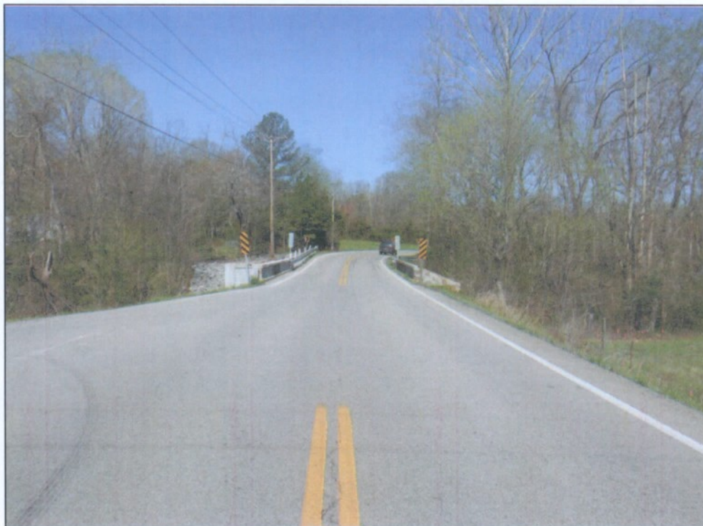
STATE ROUTE 46 WESTBOUND APPROACH TO BRIDGE
