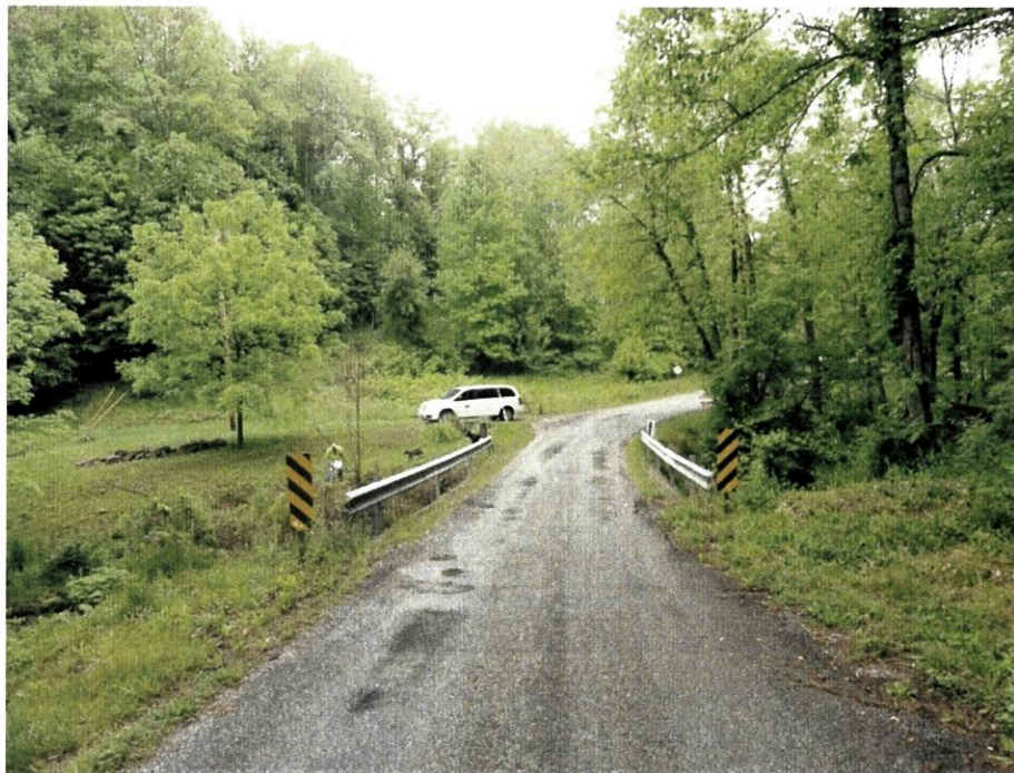
Westbound Approach (Looking West)
