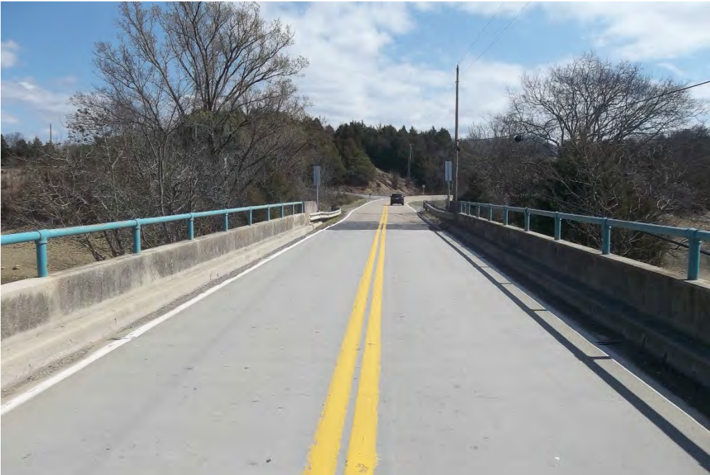
CENTER OF BRIDGE LOOKING EAST
