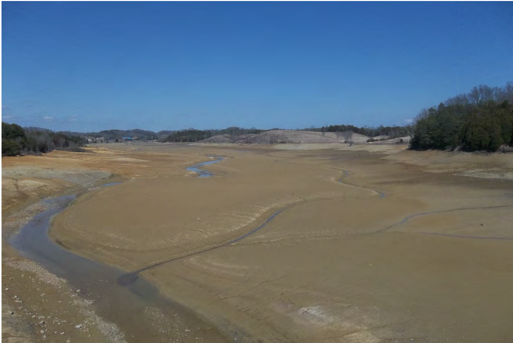
VIEW OF INLET SIDE FROM THE BRIDGE DECK
