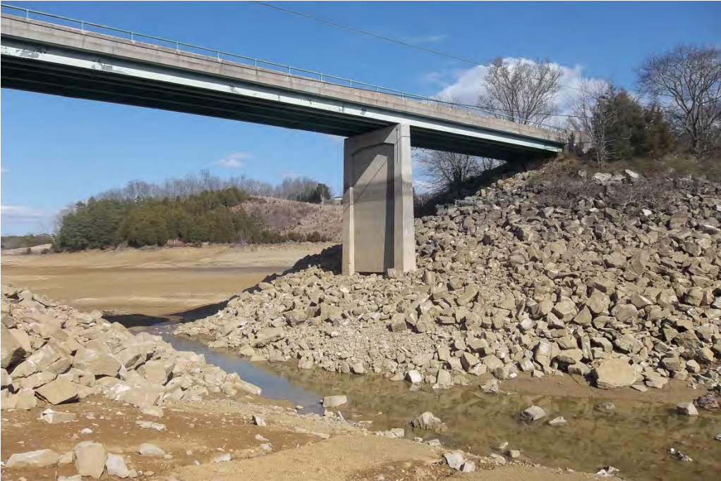
VIEW OF BRIDGE FROM THE OUTLET SIDE (LOOKING RIGHT)
