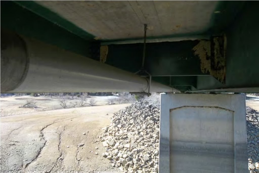
VIEW OF 6" GAS LINE LOOKING EAST UNDER THE BRIDGE DECK
