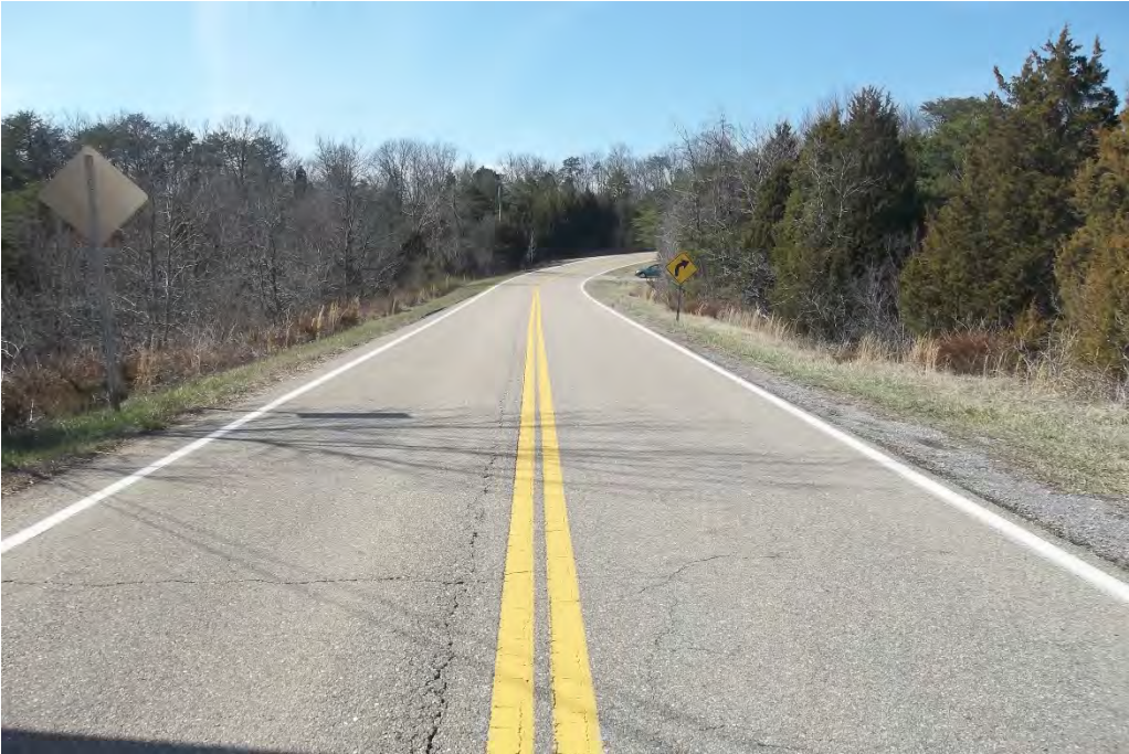
WEST APPROACH LOOKING WEST AWAY FROM THE BRIDGE
