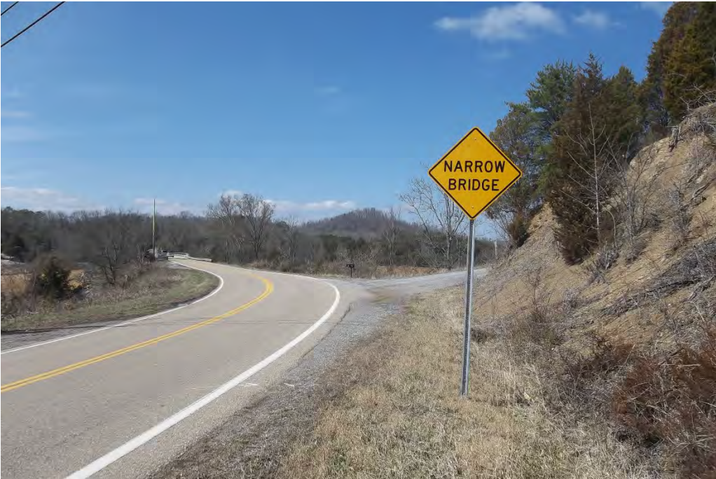
VIEW OF NARROW BRIDGE SIGN LOOKING WEST (EAST OF BRIDGE)
