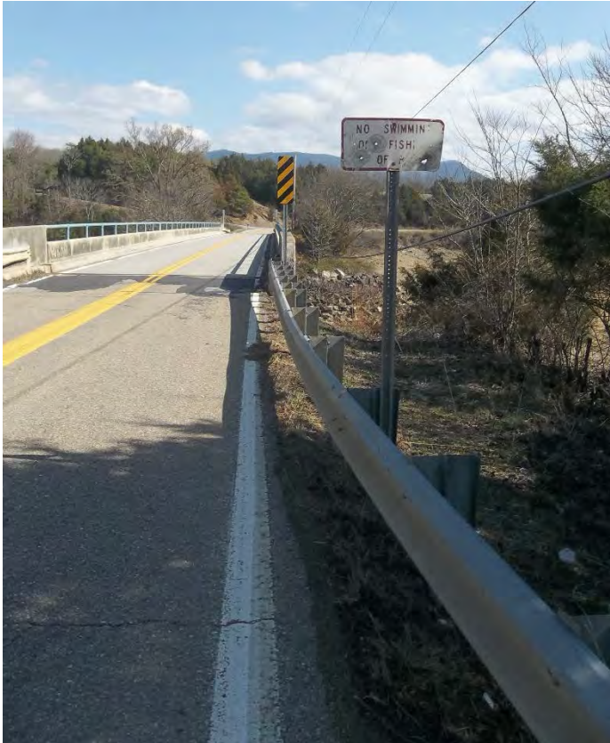
VIEW OF NO SWIMMING OR FISHING SIGN LOOKING EAST (WEST OF BRIDGE)
