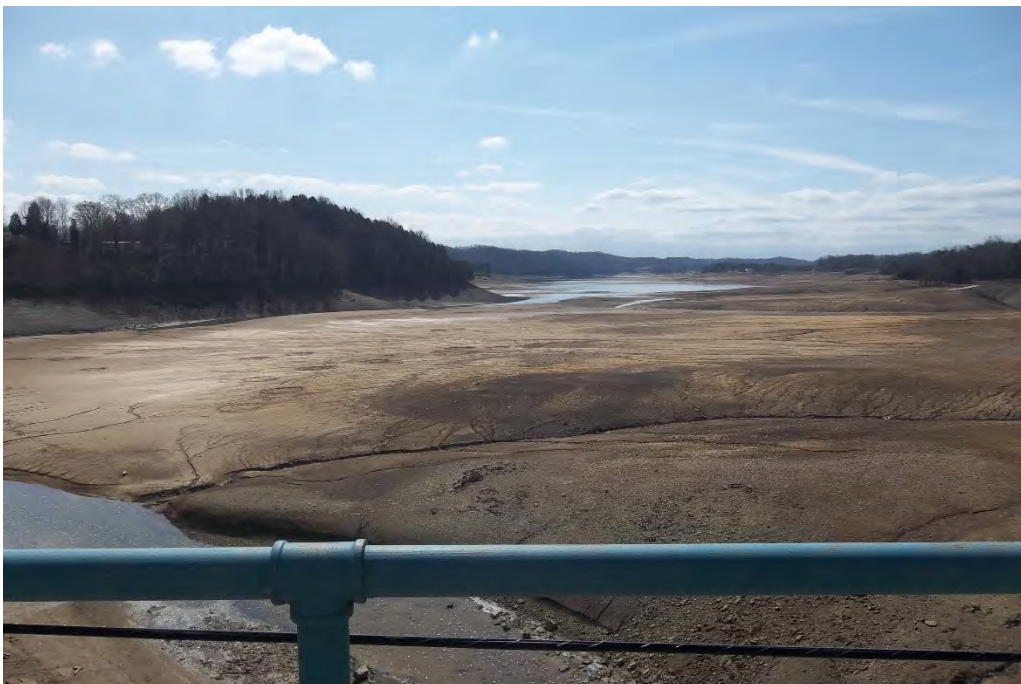
VIEW OF OUTLET SIDE FROM THE BRIDGE DECK
