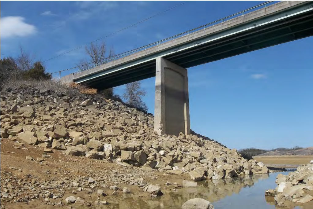
VIEW OF BRIDGE FROM THE OUTLET SIDE (LOOKING LEFT)
