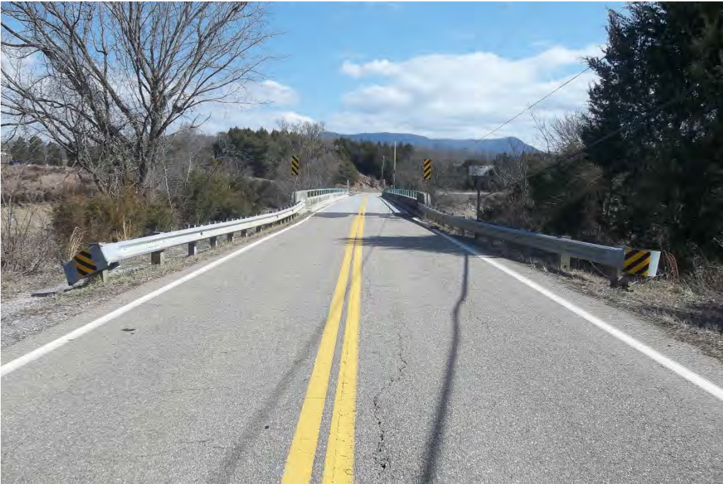
WEST APPROACH LOOKING EAST TOWARDS THE BRIDGE
