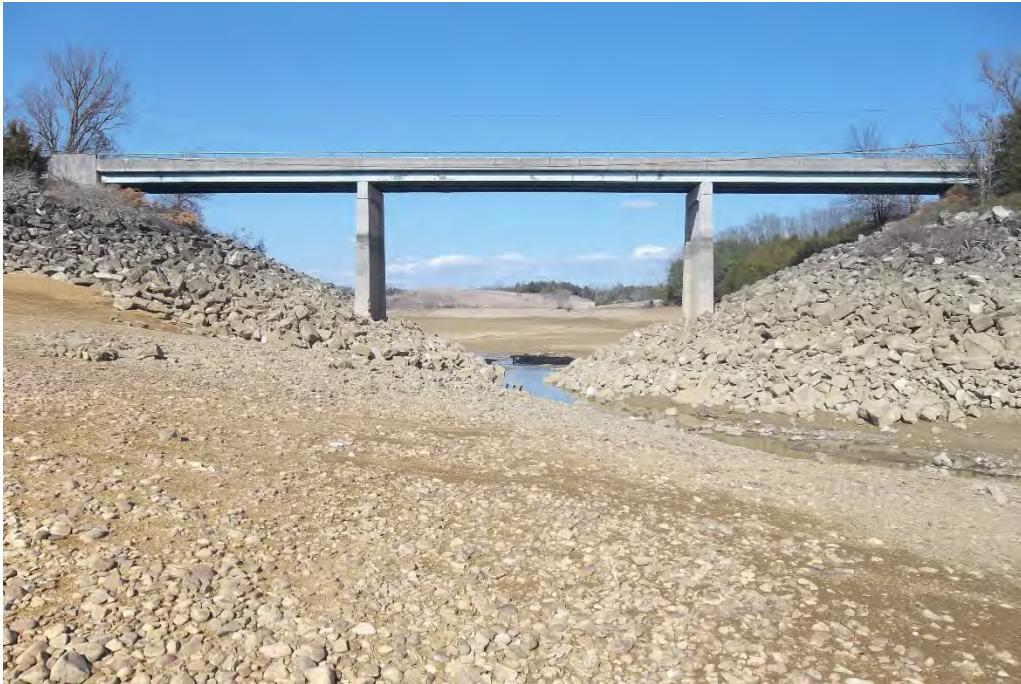
OUTLET SIDE LOOKING NORTH TOWARDS THE BRIDGE
