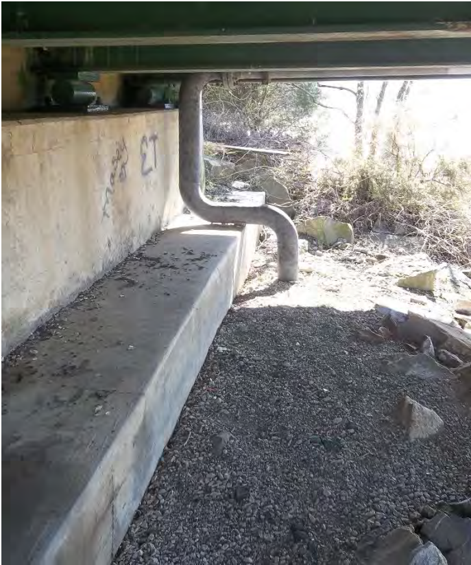
VIEW OF 6" GAS LINE LOOKING SOUTH UNDER THE BRIDGE DECK
