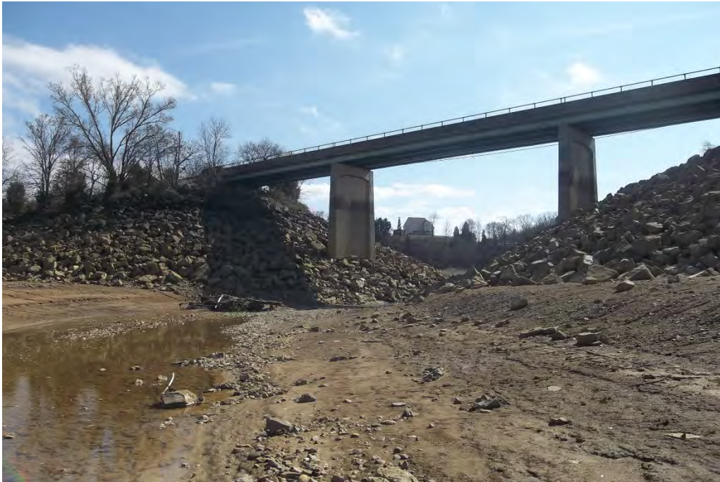
INLET SIDE LOOKING SOUTH TOWARDS THE BRIDGE
