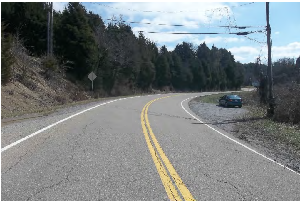
EAST APPROACH LOOKING EAST AWAY FROM THE BRIDGE
