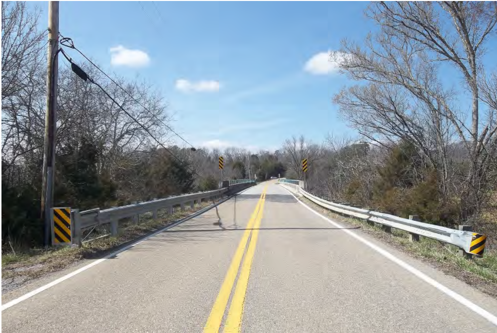
EAST APPROACH LOOKING WEST TOWARDS THE BRIDGE
