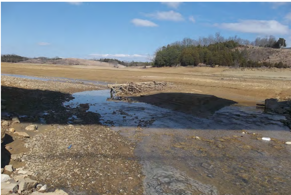
INLET SIDE LOOKING NORTH AWAY FROM THE BRIDGE
