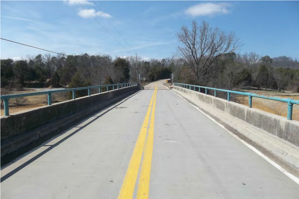
CENTER OF BRIDGE LOOKING WEST
