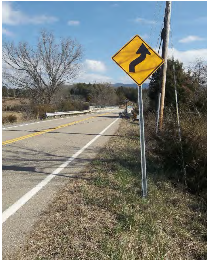
VIEW OF REVERSE CURVE SIGN LOOKING EAST (WEST OF BRIDGE)
