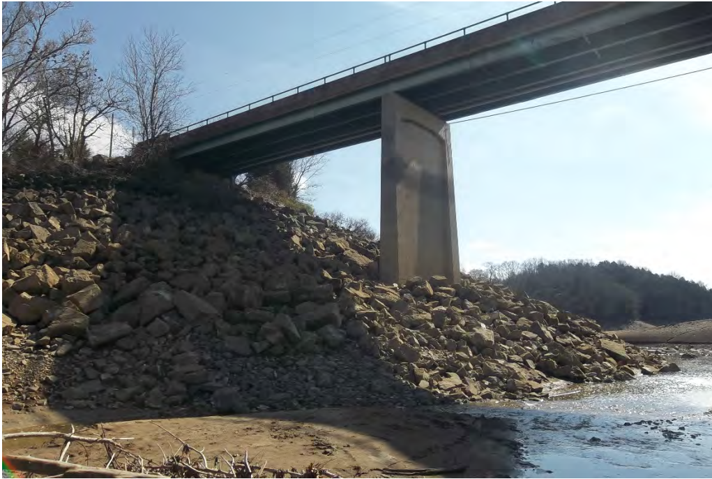
VIEW OF BRIDGE FROM THE INLET SIDE (LOOKING LEFT)
