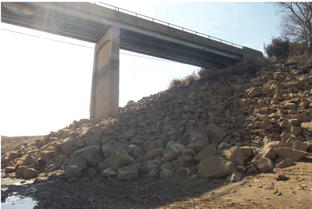
VIEW OF BRIDGE FROM THE INLET SIDE (LOOKING RIGHT)
