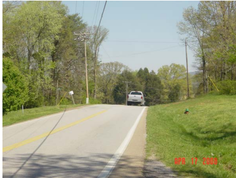
Vertical curve at Griffin Lane, looking east
