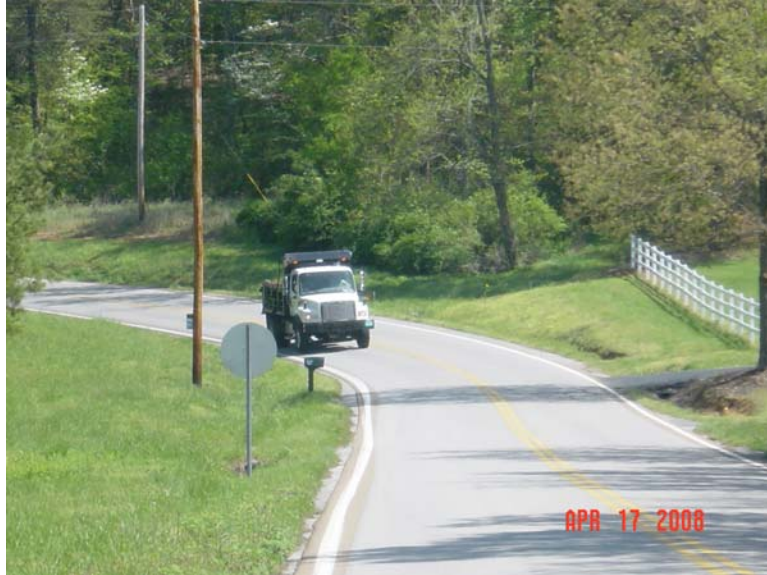
Curve at LM 18.95, looking east
