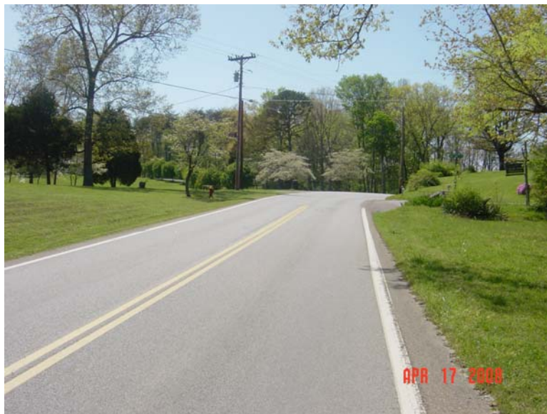
Vertical curve at Mail Loop Road East, looking west
