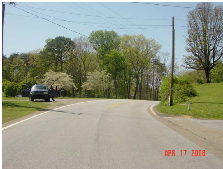
Horizontal curve at Mail Loop Road East, looking west
