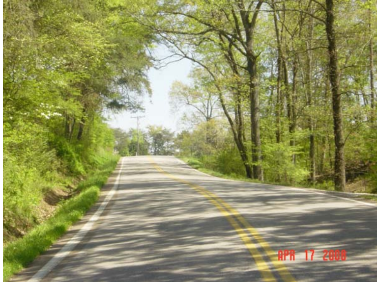
Vertical curve at Mail Loop Road East, looking east
