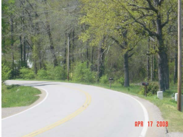
Horizontal curve at Log Mile 17.33, looking west
