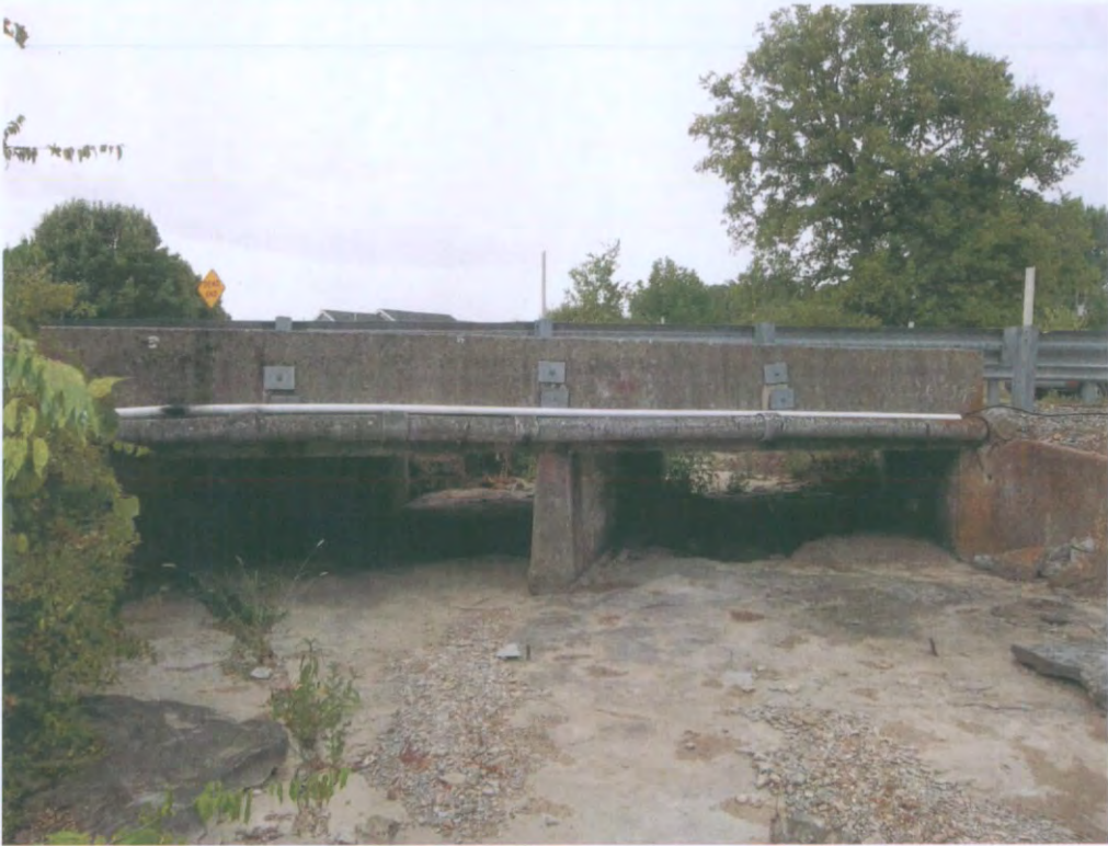
OUTLET SIDE LOOKING NORTH TOWARDS THE BRIDGE
