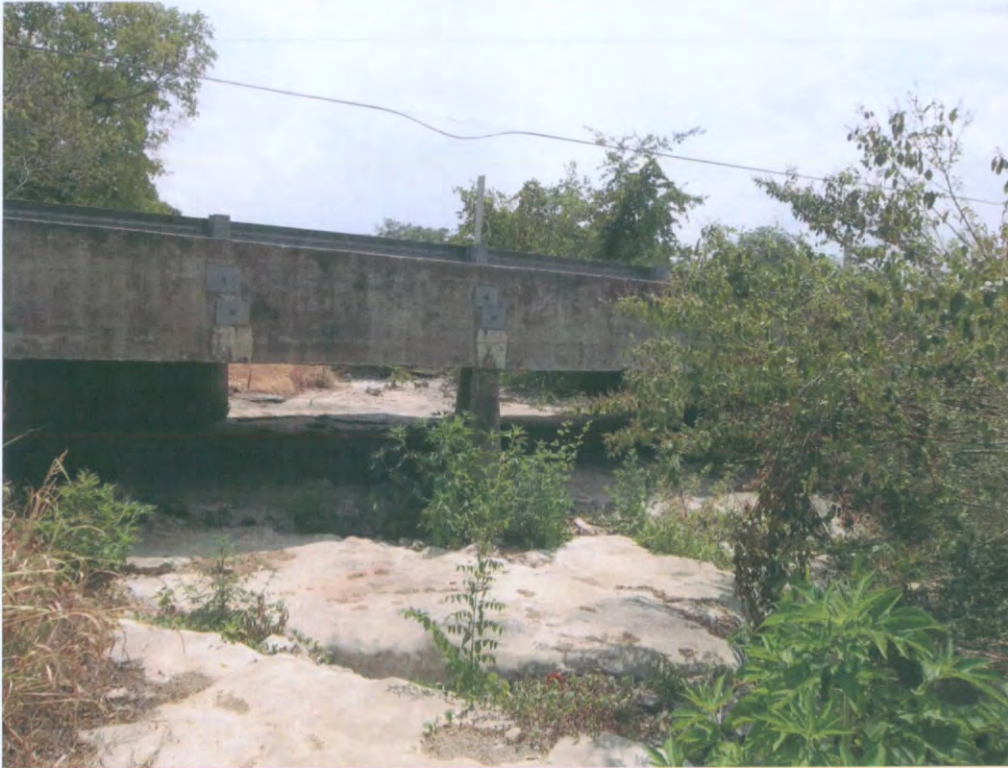
INLET SIDE LOOKING SOUTH TOWARDS THE BRIDGE
