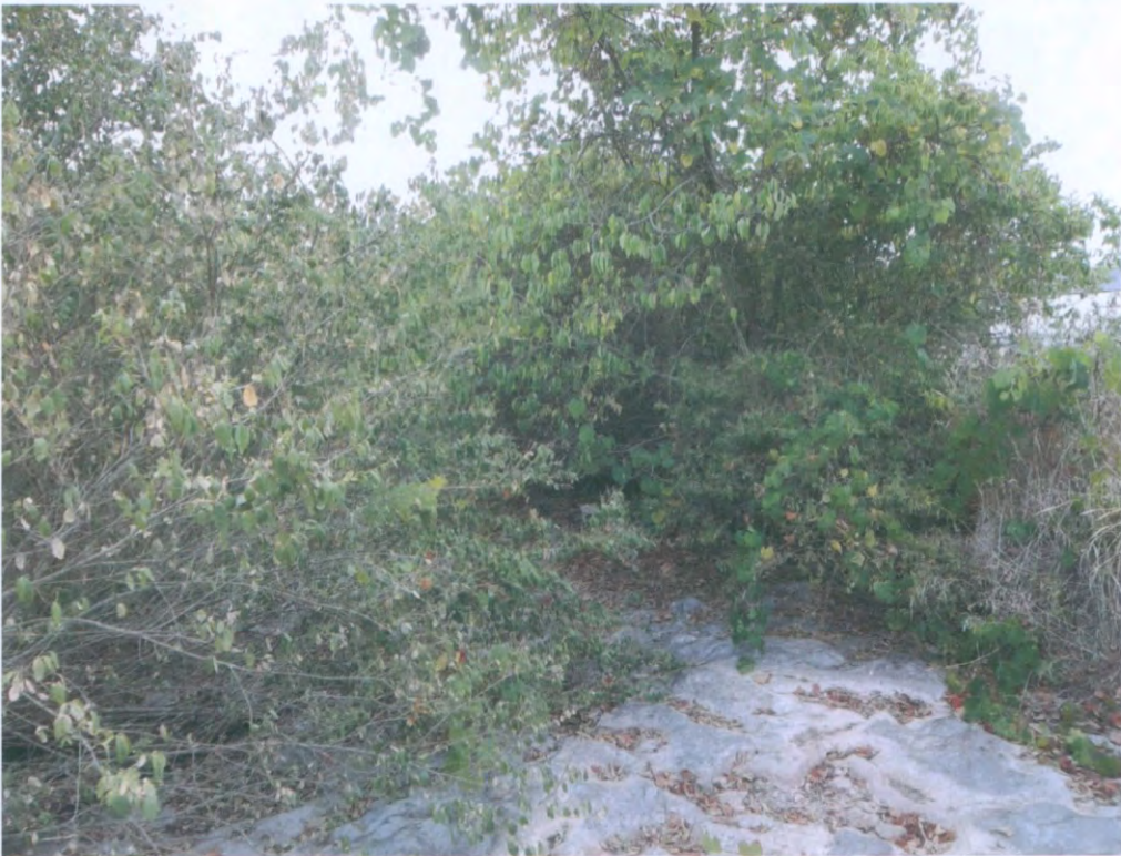
OUTLET SIDE LOOKING SOUTH AWAY FROM THE BRIDGE
