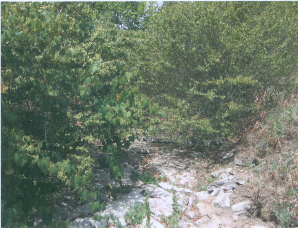
INLET SIDE LOOKING NORTH AWAY FROM THE BRIDGE
