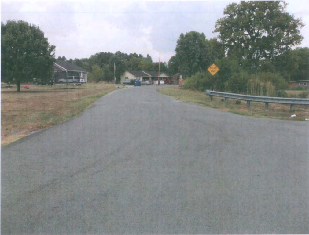
WEST APPROACH LOOKING NORTH AT APRIL LANE
