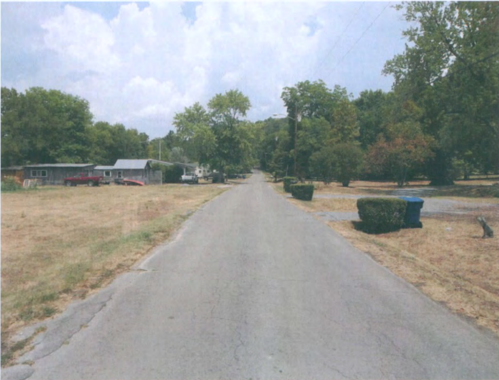
EAST APPROACH LOOKING EAST AWAY FROM THE BRIDGE
