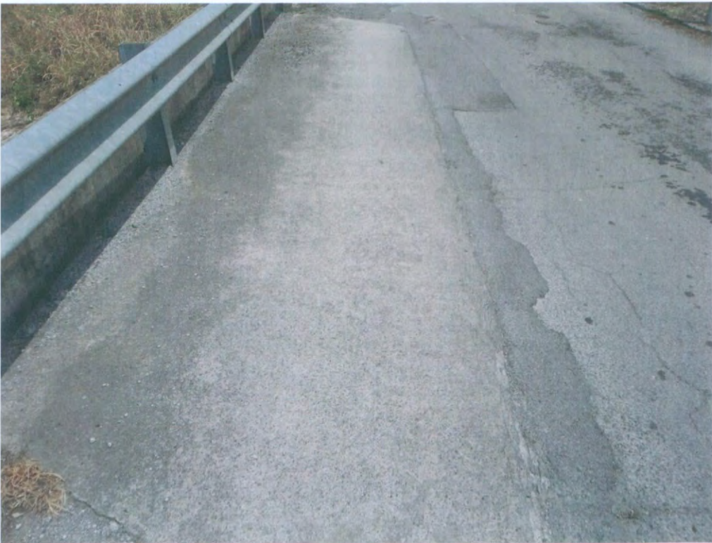
VIEW OF PREVIOUSLY REPAIRED SECTION
