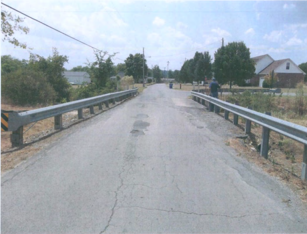
EAST APPROACH LOOKING WEST TOWARDS THE BRIDGE
