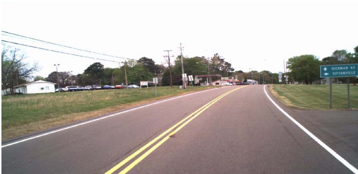
Existing State Route 5 12' travel lane with 2' shoulders
