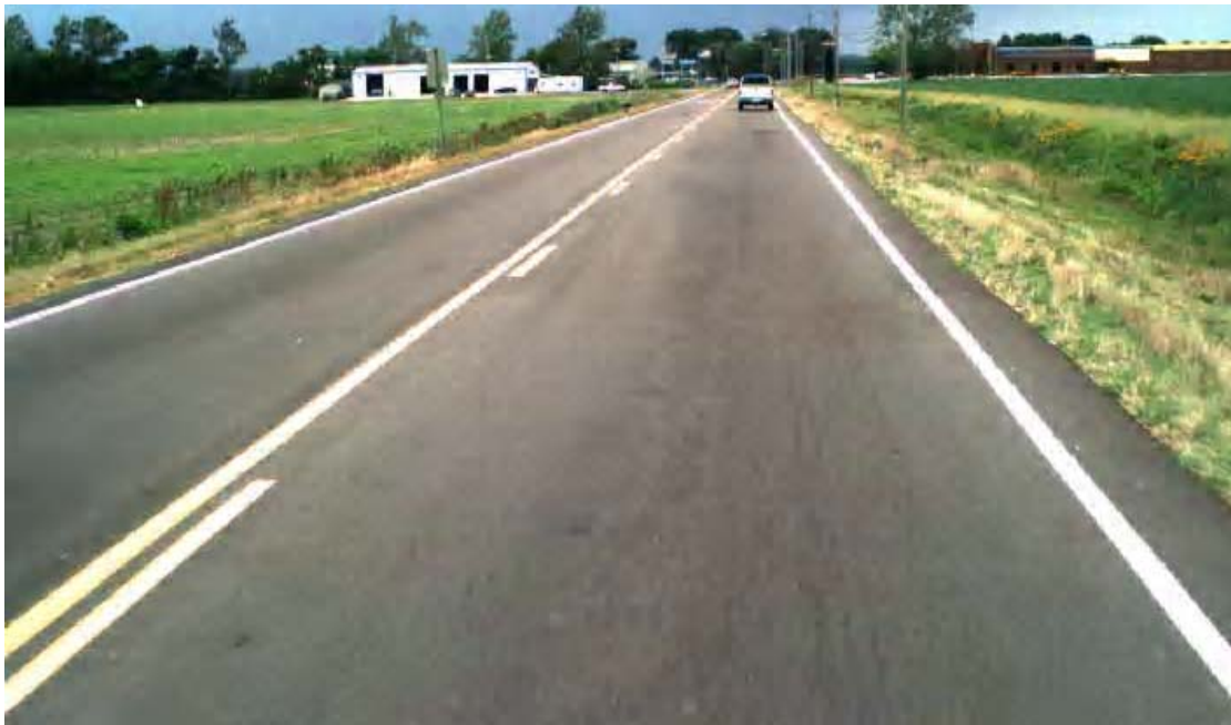
Existing State Route 5 12' travel lane with 2' shoulders
