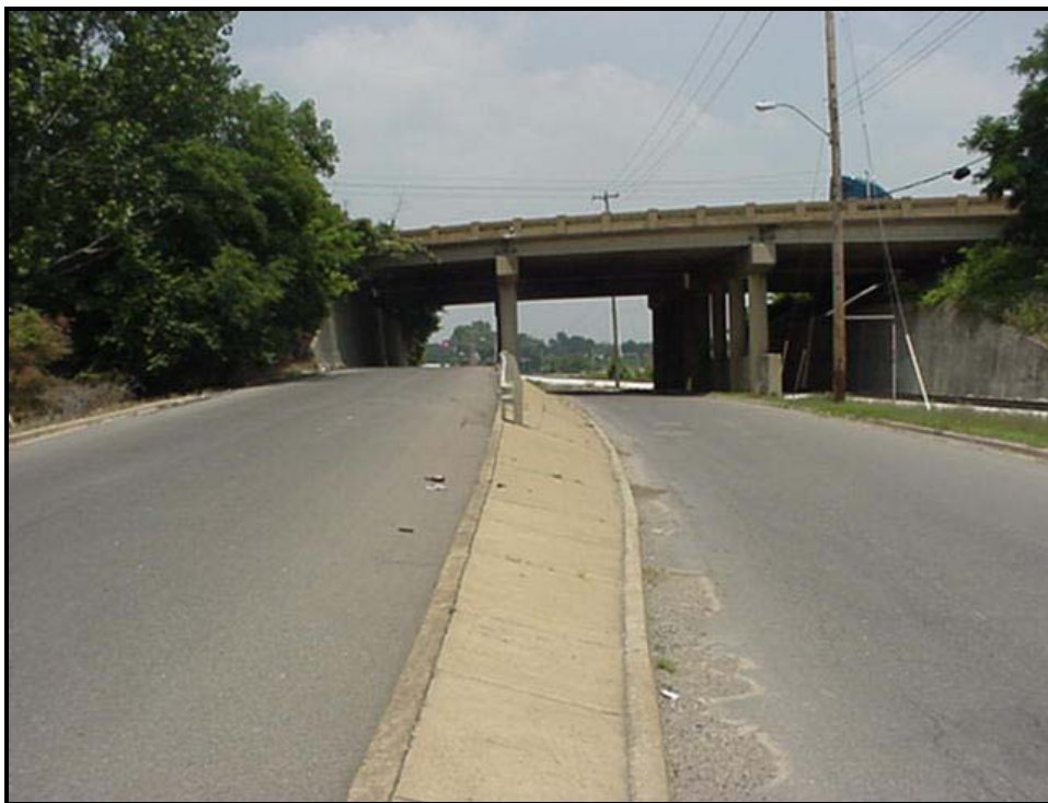
Photo 4: Riverport Road West of I-55 towards Mallory Avenue
