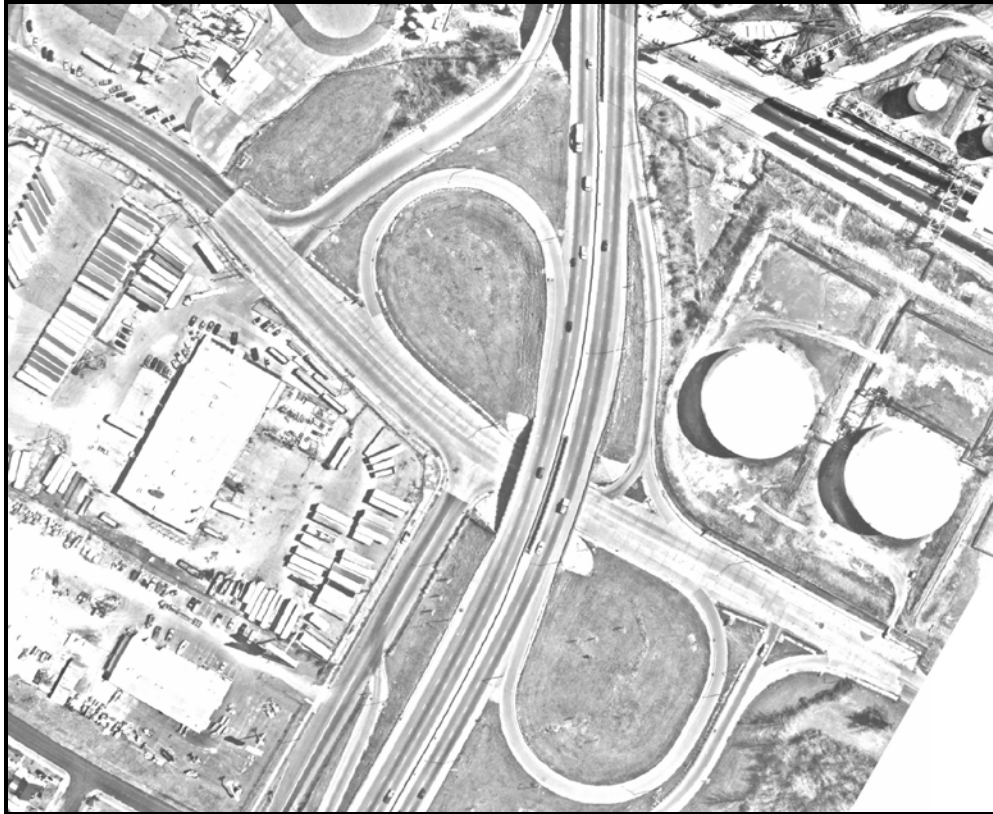
Photo 1: Aerial picture of the I-55 and Mallory Avenue Interchange
