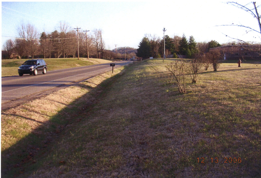
Roadside ditch along east side of northbound approach of SR-106
