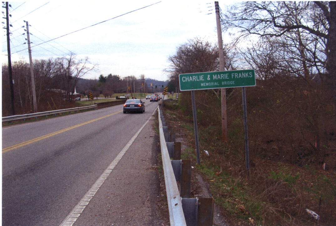
Existing bridge over Cartwright Creek (Southbound SR-106)
