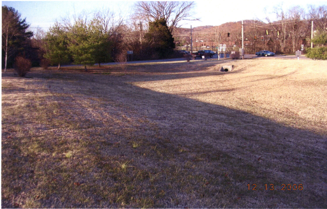
Detention area adjacent to Intersection of SR-106 and SR-46.
