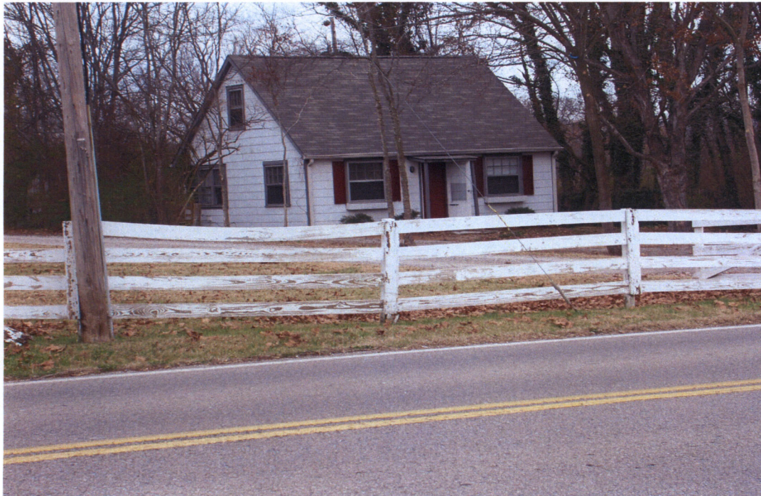
Residential home located on SR-46 near intersection with SR-106.
