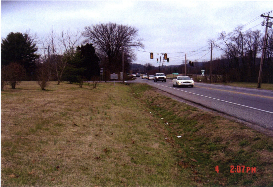
Looking north along SR-106 toward intersection.
