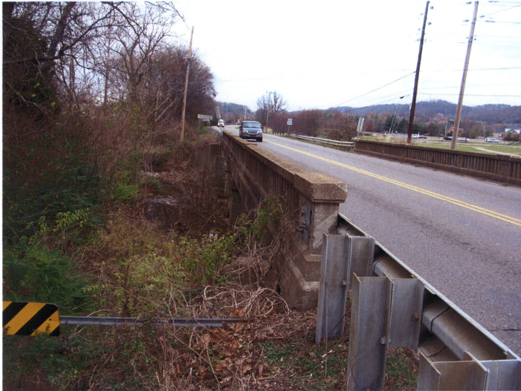
Existing bridge over Cartwright Creek (Northbound SR-106)
