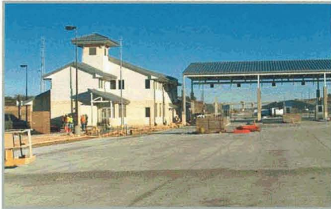
ABOVE: Loop 1 Extension, Mainlane Toll Plaza, January 2006
