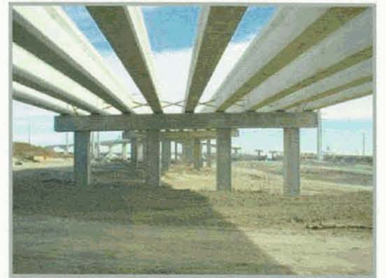
ABOVE: Ramp Construction, SH 45N, Section 6, January 2006
