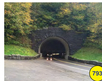
Stone tunnel headwall (+)
