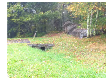
Stone culvert at Deep Creek Valley Overlook 2 (+)
