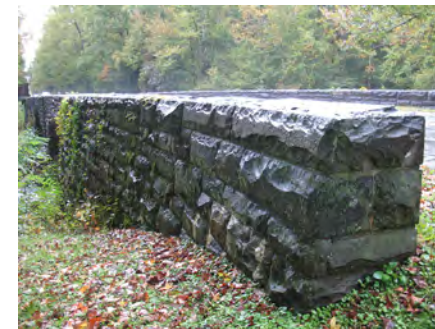
Stone arch bridge (+)
