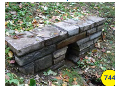
Stone headwall/culvert (+)
