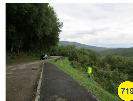
Asphalt walkway and vegetation at Carlos Campbell Overlook North (-)
