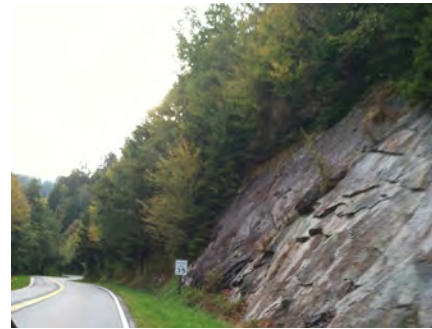
Rock face on the right (SB) (+)
