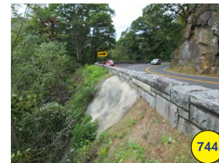
Stone guard wall with concrete repair (-)
