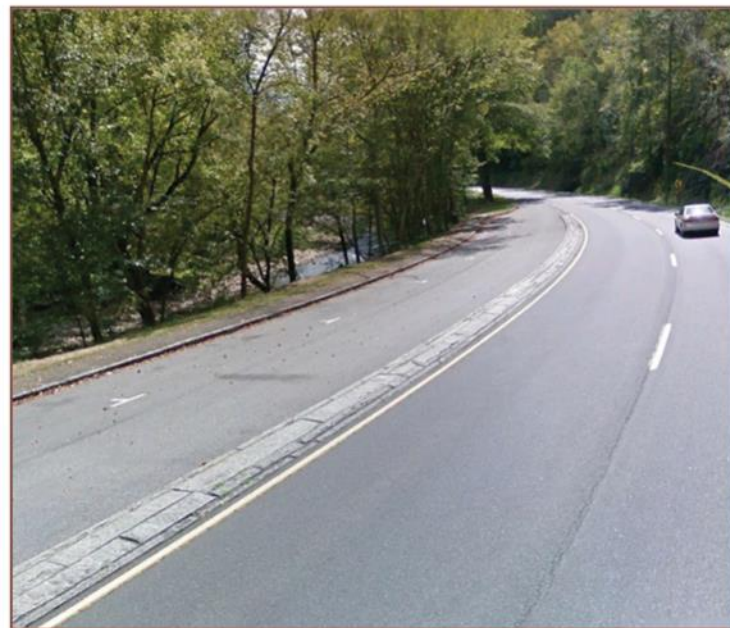
Stone safety island on the Gatlinburg Spur route
