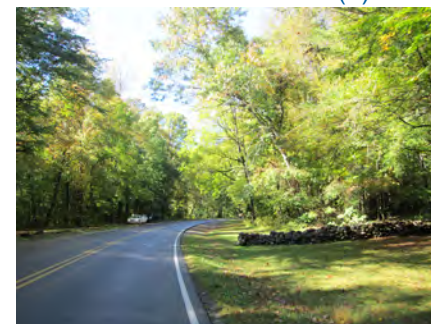
Stone wall at Cherokee park entrance (+)
