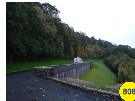
Retaining wall/guard wall at pull off (-)
