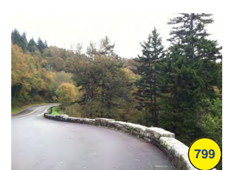
Stone wall at pull off (+)
