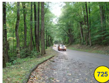
Pull off with stone curbing and asphalt (o)
