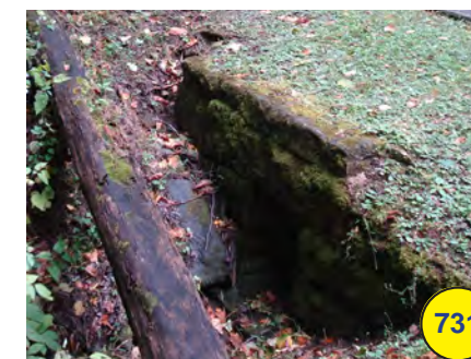
Stone headwall/culvert (o)
