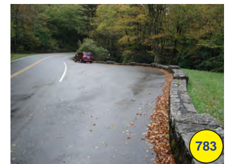
Asphalt pull off with stone wall and limited striping (+)
