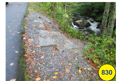
Precarious steps to stream (-)
