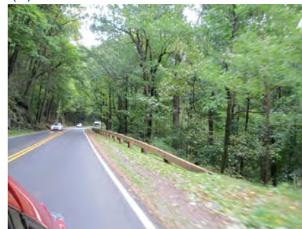
Wooden guardrail (o)
