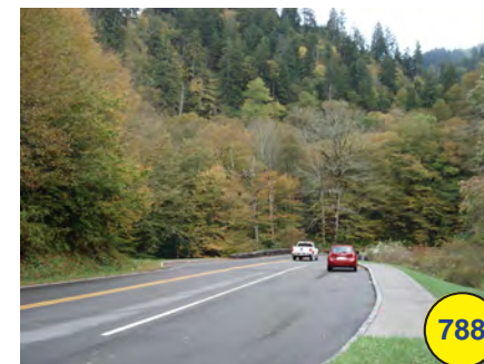
Pull off at stone bridge (+)
