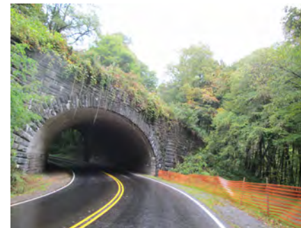
Construction fence at The Loop tunnel (-)
