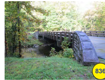
Stone bridge with wood guardrail at Smokemont (+)
