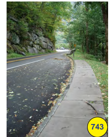
Pull off with concrete sidewalk (o)
