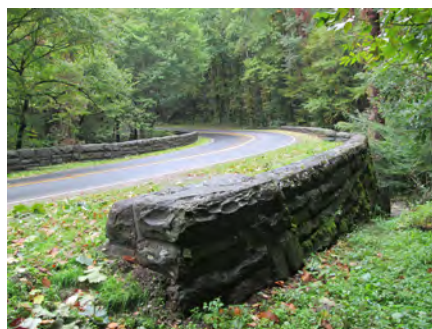
Stone arch bridge over the West Prong of the Little Pigeon River (+)
