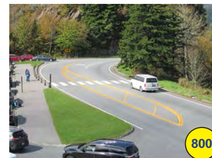
Pedestrian and vehicle conflict at crossing to the Appalachian Trail (-)
