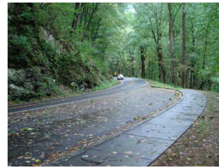
Pull off with concrete sidewalk (o)
