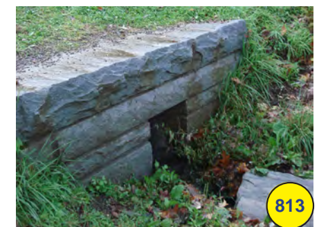
Stone headwall/culvert (o)
