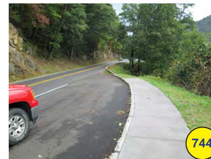
Asphalt overlook with stone and concrete at Chimney Tops Overlook (o)
