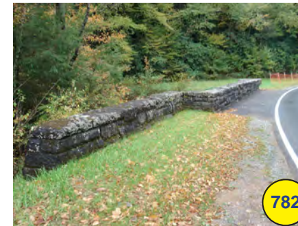
Stone bridge and wall (+)
