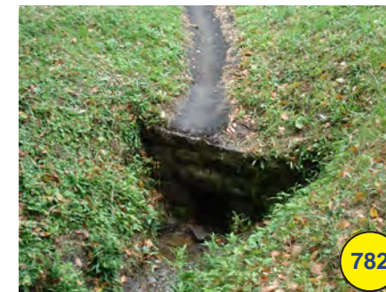
Culvert with shallow asphalt swale (-)
