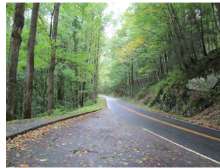
Asphalt with stone curbing pull off (o)
