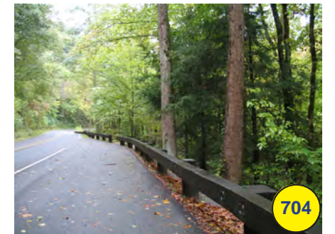
704 Pull off and wood guard rail (o)
