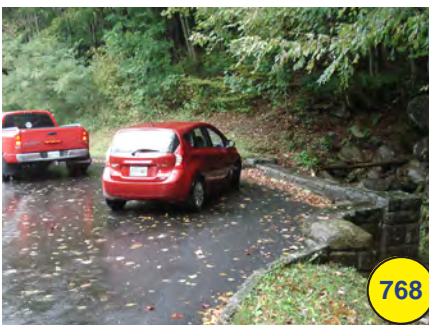
Stone headwall at pull off (+)
