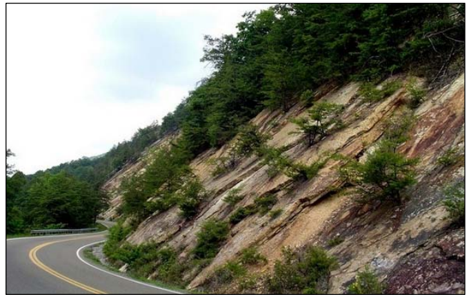
Figure 1. Rock slope on State Route 70 in Hawkins County
