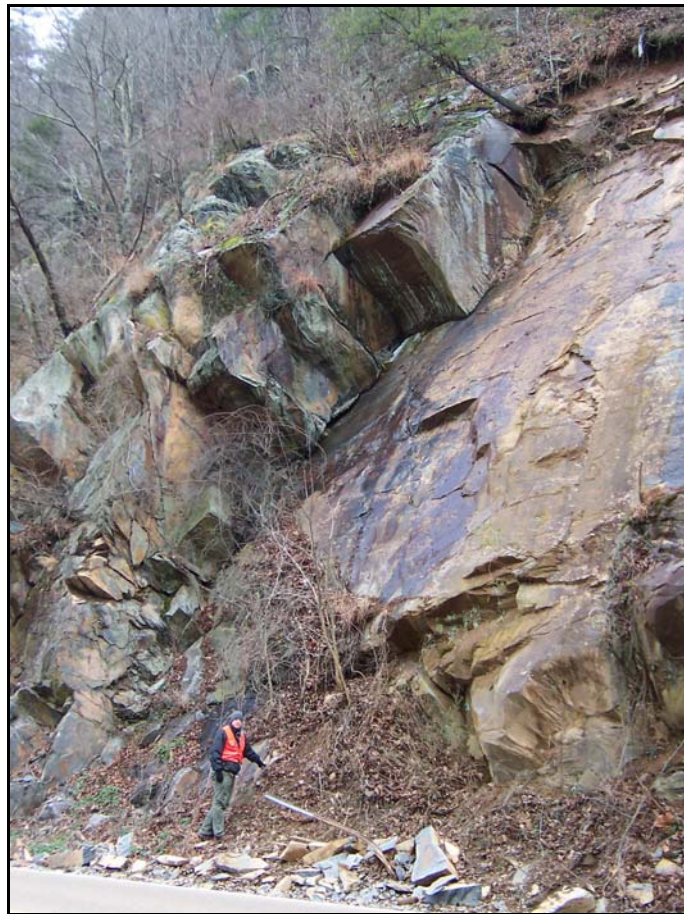
Figure 2-21: Planar Rockfall Mode: Polk County SR040, mile 14.0 left Overall Score – 512
