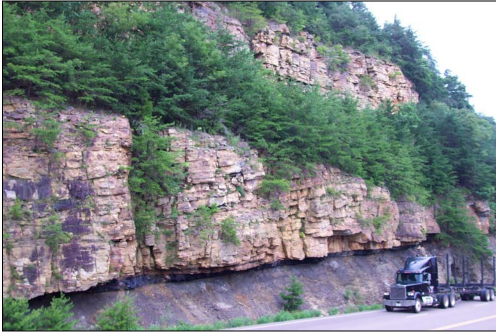
Figure 2-11: Toppling and Differential Weathering Rockfall Modes: Sequatchie County SR008, mile 21.2 right
