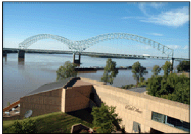
Hernando DeSoto Bridge Source: City of Memphis website
