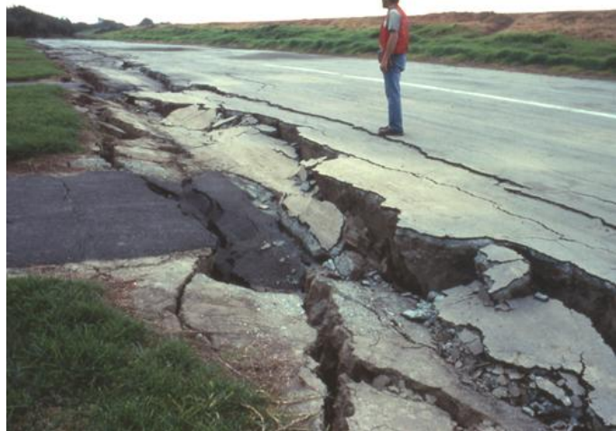
Above: Road damaged by lateral spreading near Pajaro River, 1989 Loma Prieta earthquake.
