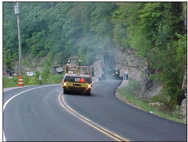
DeKalb County - SR 26 – Binder (BM-2) Placement
