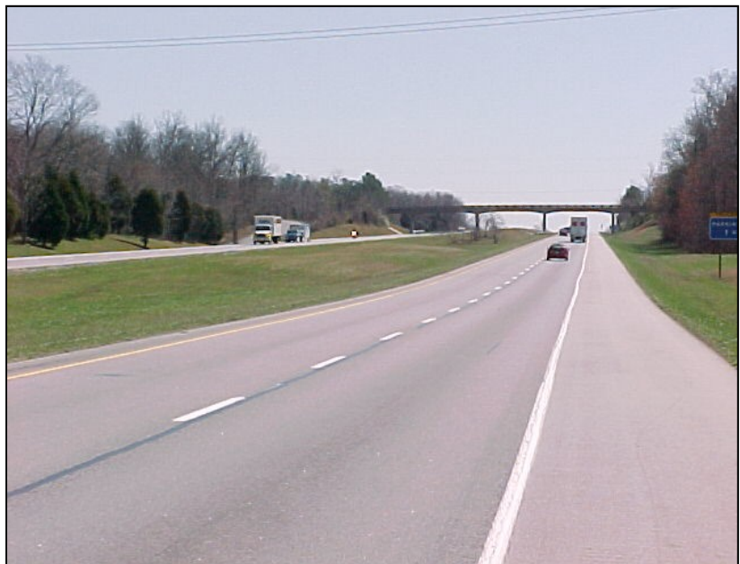
Centerline joint sealed
