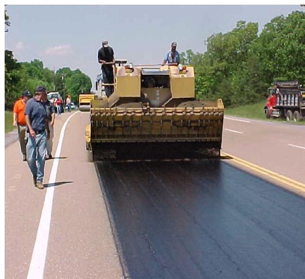
Aggregate applied to asphalt
