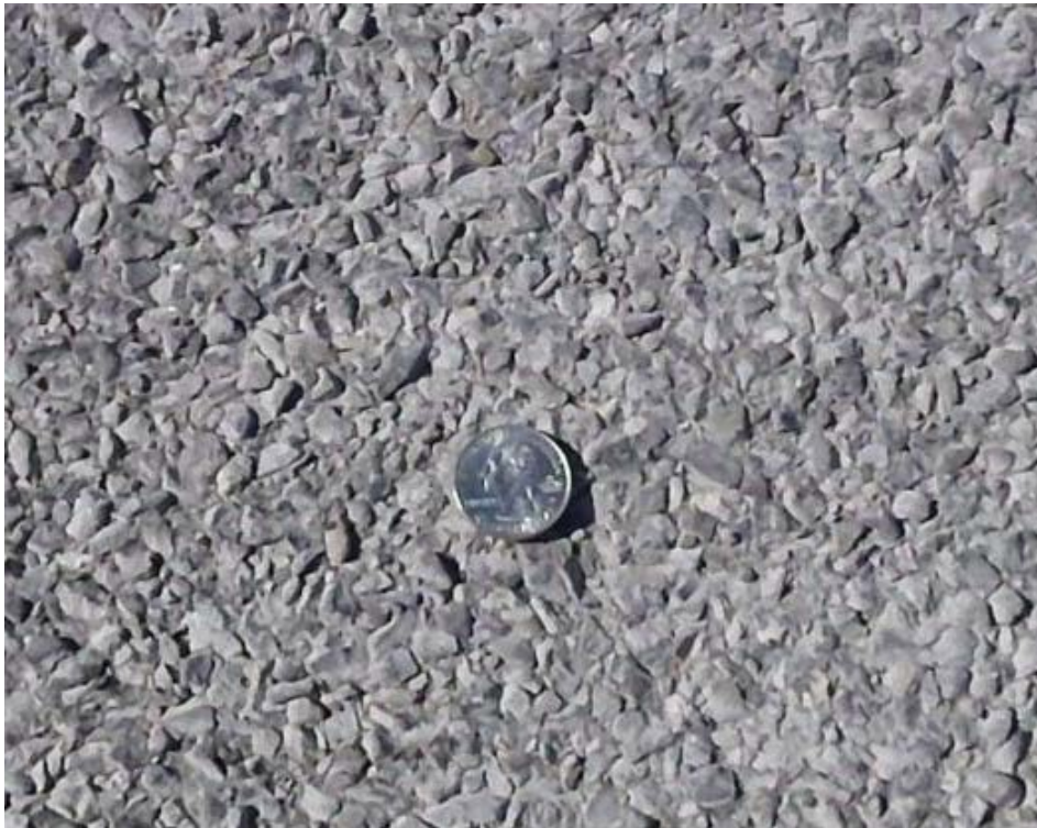
Chip Seal prior to Microsurfacing Lift being placed
