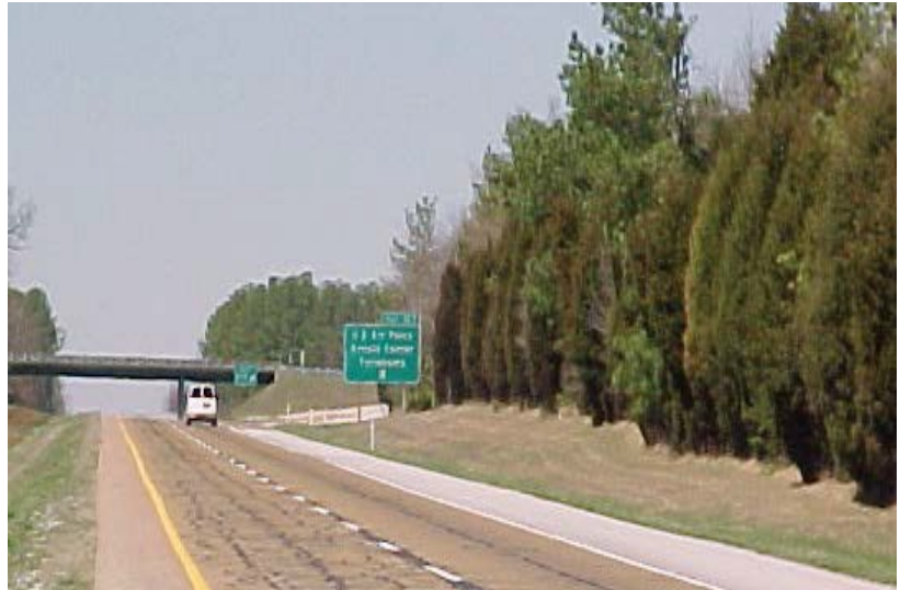
Excessive crack sealing of secondary cracks creating safety concerns
