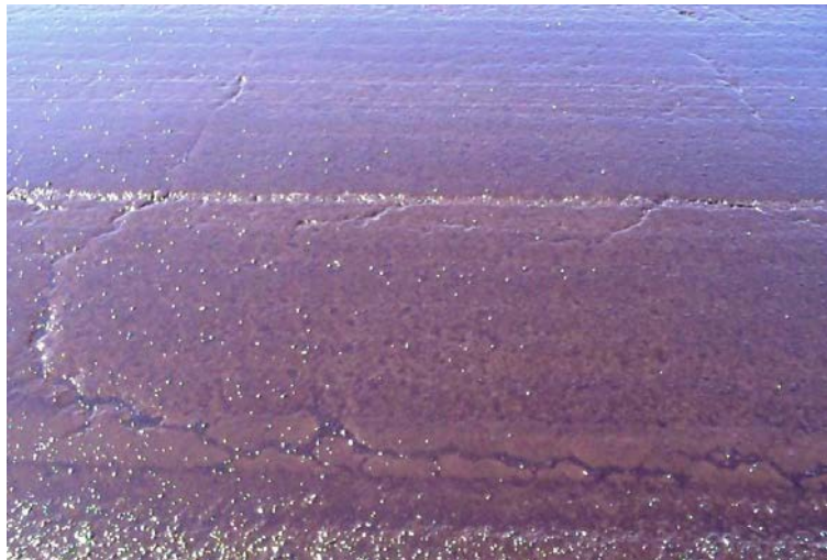
CRS2P Emulsion filling cracks prior to aggregate placement
