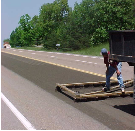
Brooming of aggregate cover material
