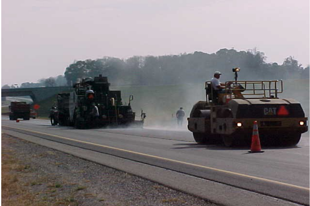
SR 111 - White County - 1-1/4" "D" Mix with 2-foot taper on shoulders
