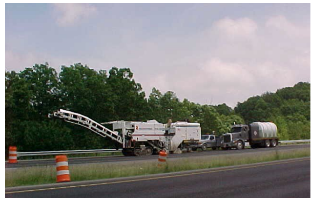
Milling Machine and Water Truck
