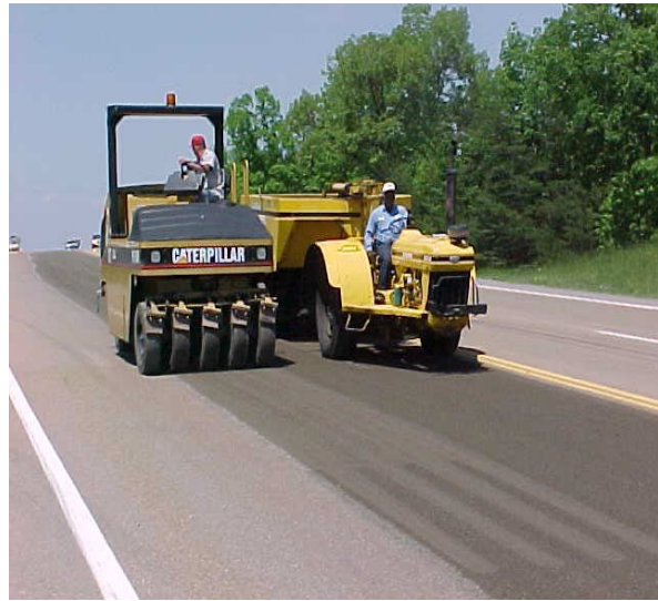
Rolling of aggregate cover material – 2 passes
