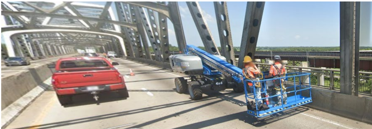
Figure II-2: Routine Maintenance on the I-55 Bridge in August 2022
