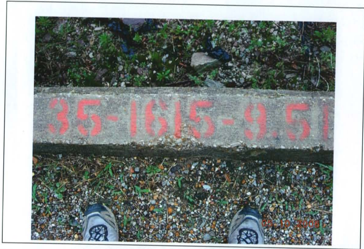
ABOVE: Bridge Location Number
