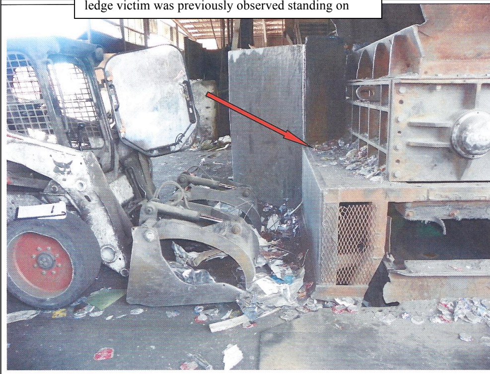
Loading of shredder where fatality occurred showing ledge victim was previously observed standing on
