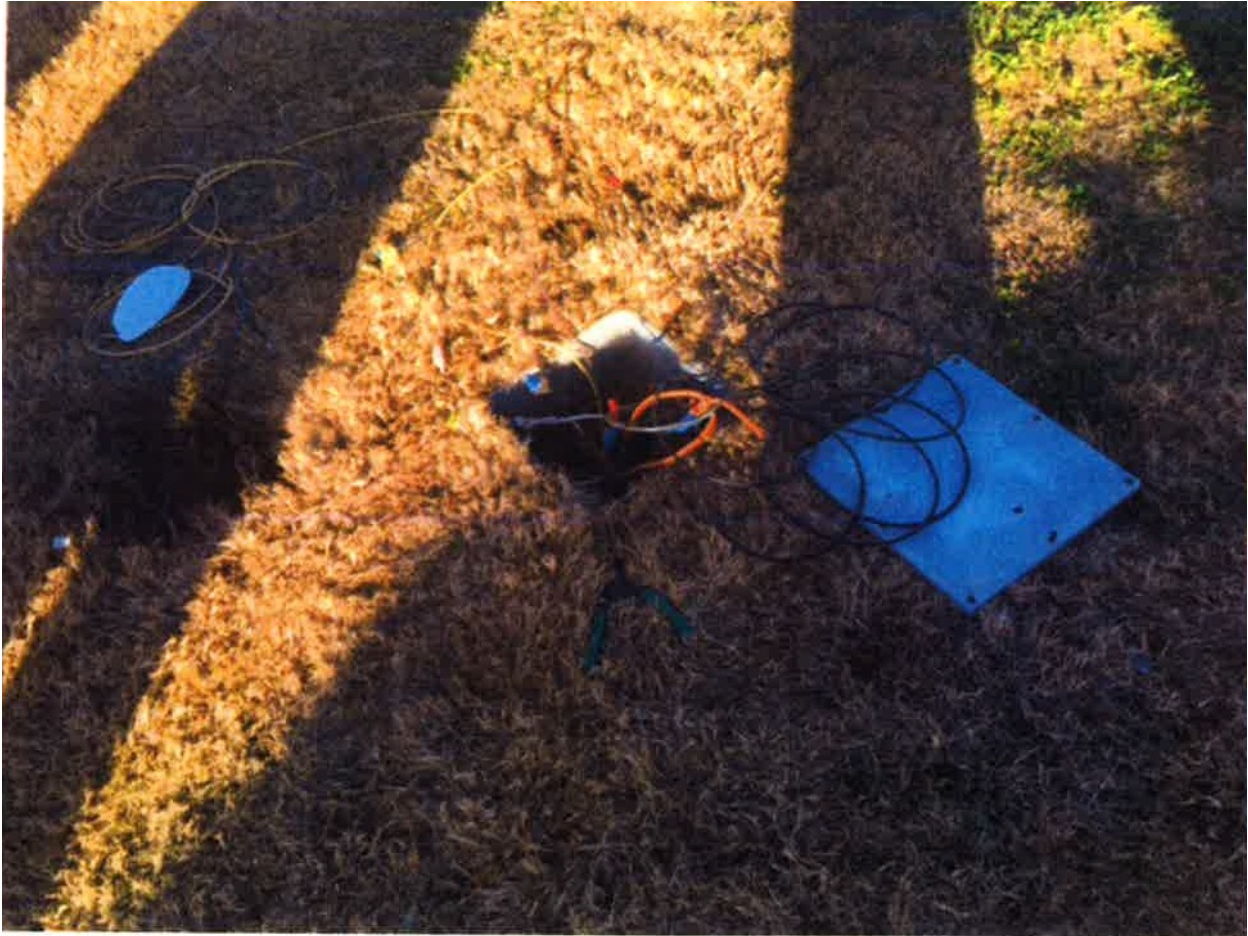
Photo 1 of 1 – Photo of junction box where victim was found.
