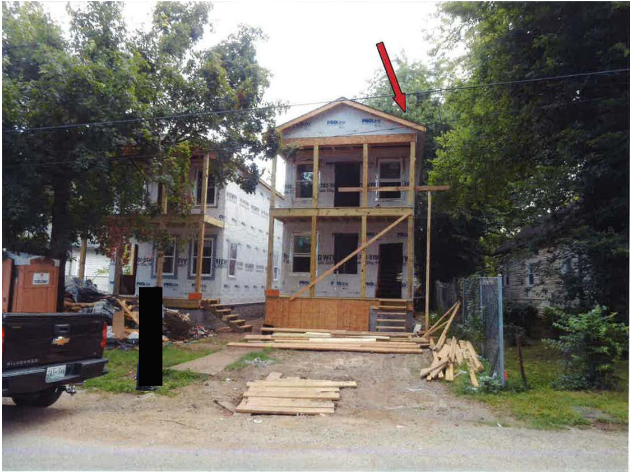
Photo 1 of 1 – Red arrow indicates where the victim fell from the 3:12 pitched residential roof to the ground below.
