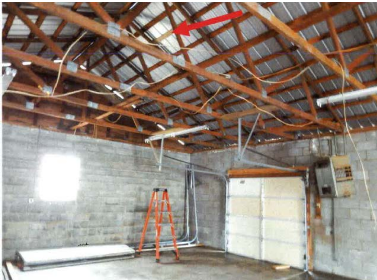
Photo 1 of 1 – Shows the area where the victim fell. The red arrow in the photo indicates the piece of lath that the victim was sitting on just before he fell. This piece of lath broke.
