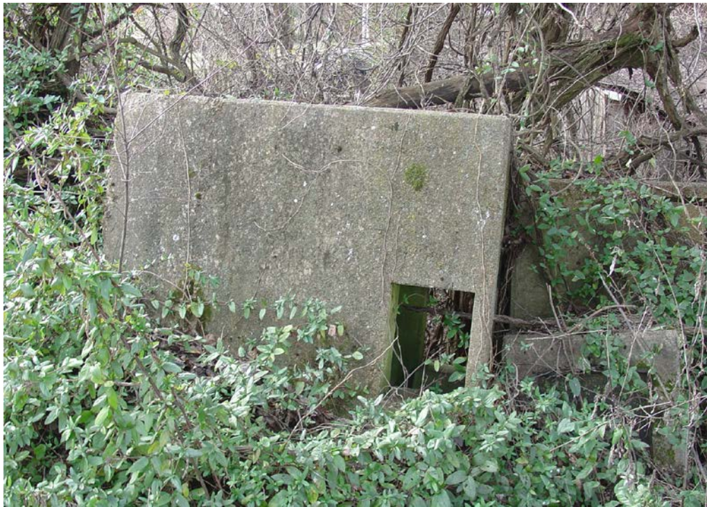
Figure 26. Concrete structure for anti-aircraft gun turret at 40LA174 (TDOA WWII image file, photo #S043).
