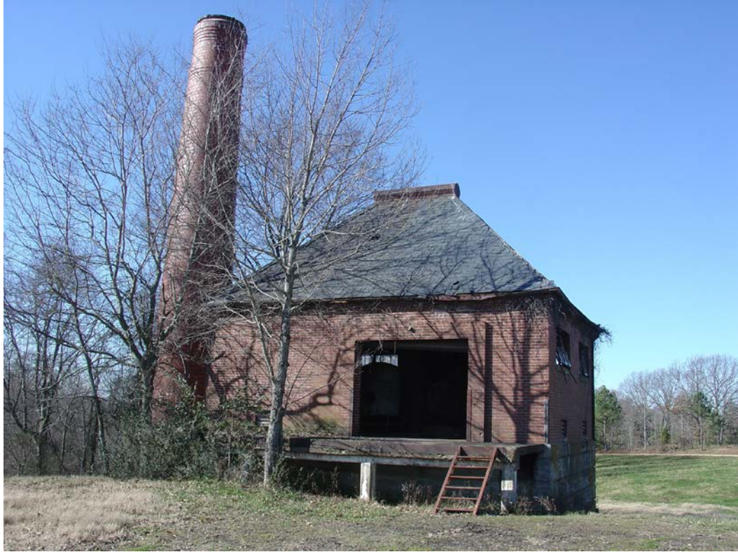
Figure 19. 2004 photo of incinerator building at Camp Tyson (TDOA WWII image file, photo #S015).
