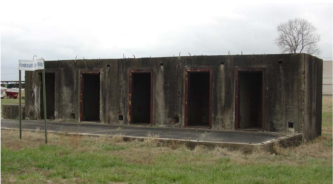
Figure 12. 2004 photo of vaults at Dyersburg Army Air Base (TDOA WWII image file, photo #S049).
