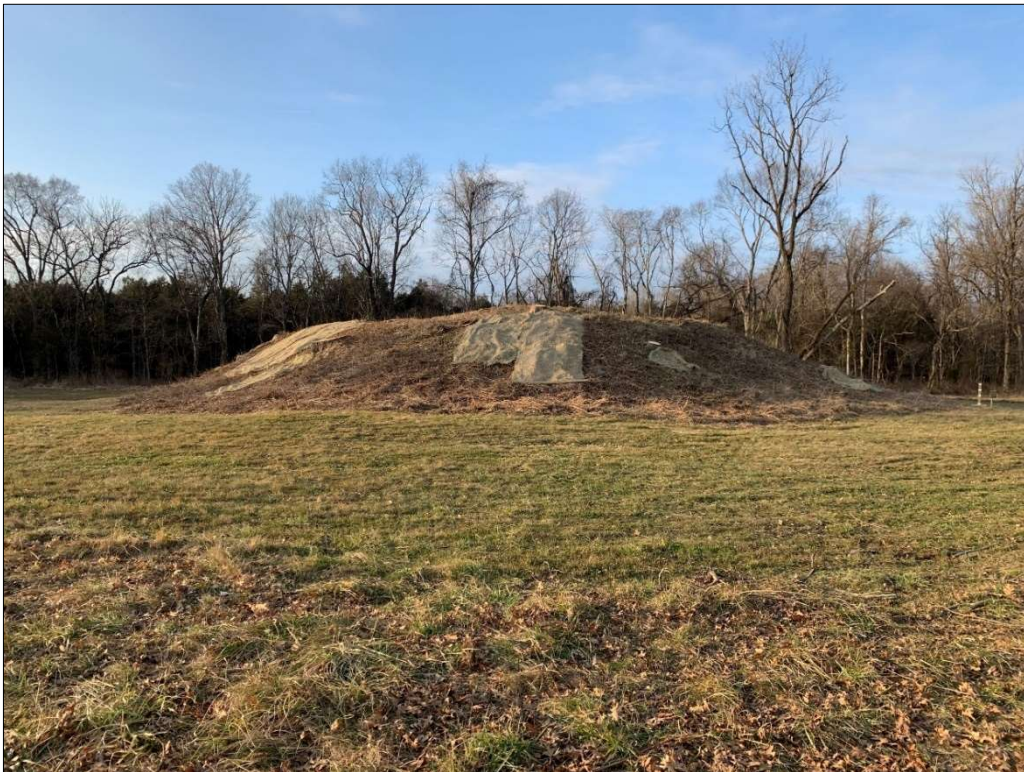
And after tree removal, showing straw mats used to prevent erosion.
