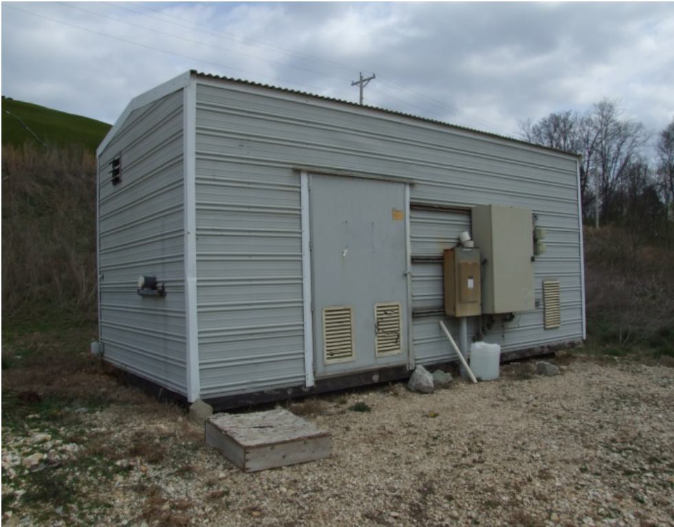
Gas Management Building
