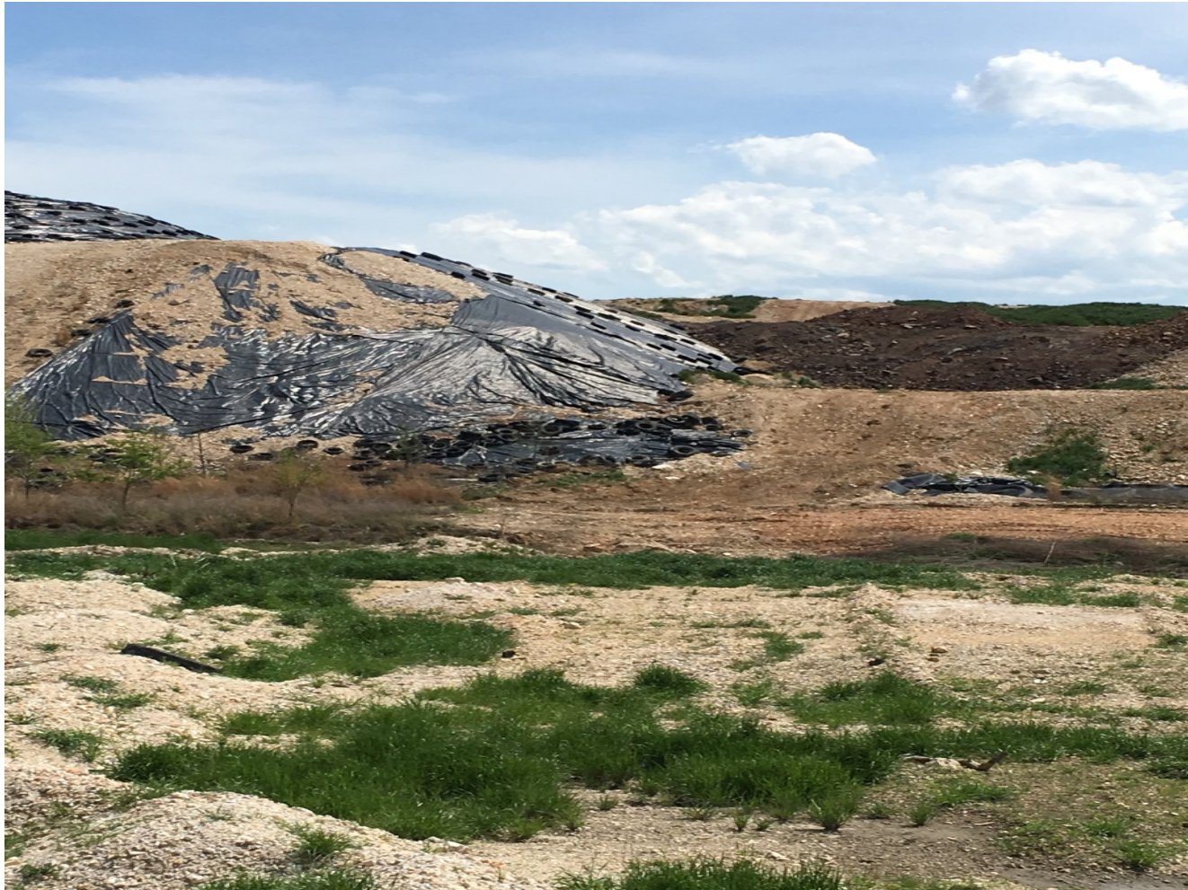
Clay Placement on APWC – View From Ground
