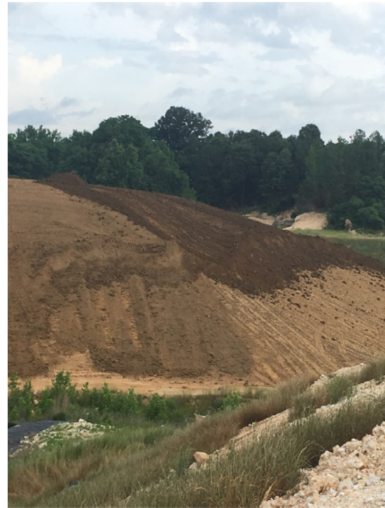
Top Soil Placement
