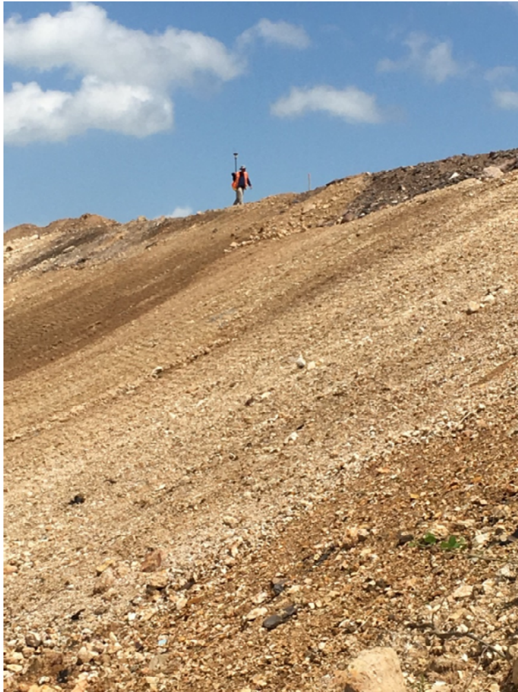
Surveying Existing Grades
