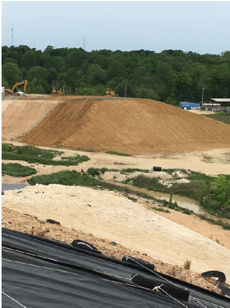
Clay Placement Complete
