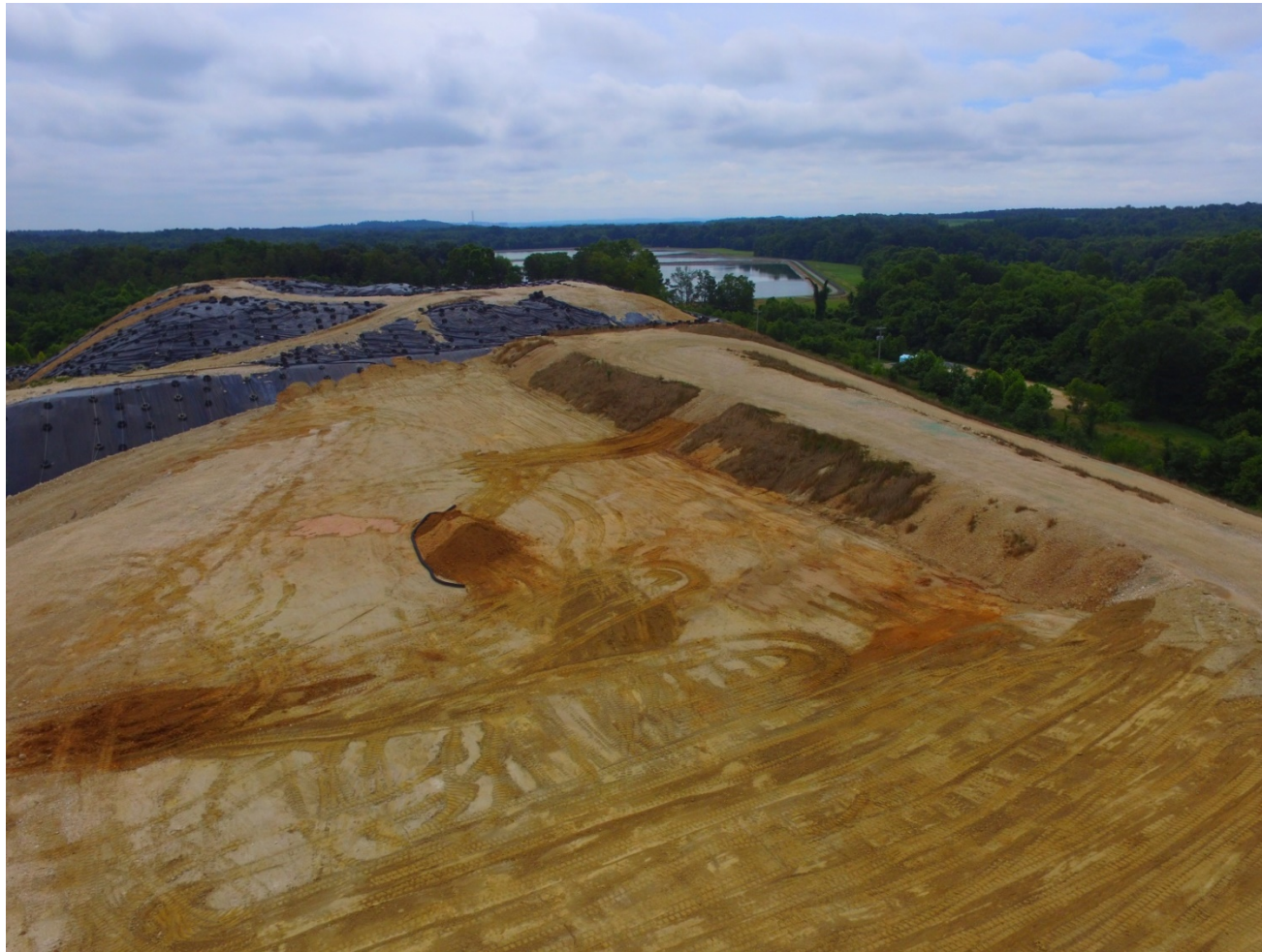
Drone Close-Up Of Clay Placement Areas
