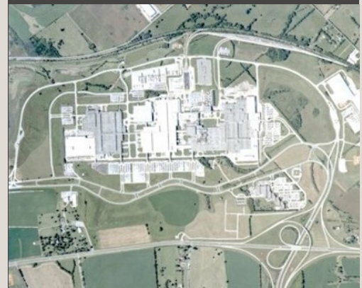
Bird's-eye view of the Spring Hill General Motors facility.
