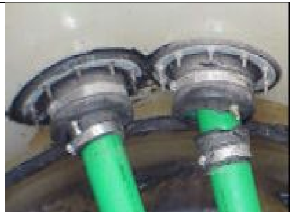
2. Environ Geo-Flex Test Boot attached to penetration fitting; test boot on right
