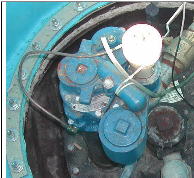
Correct MLLD vent tube installation on FE Petro submersible pump (bottom tank port).
