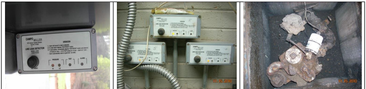
Campo/Miller LS-300 Pressure Transducer ELLD
