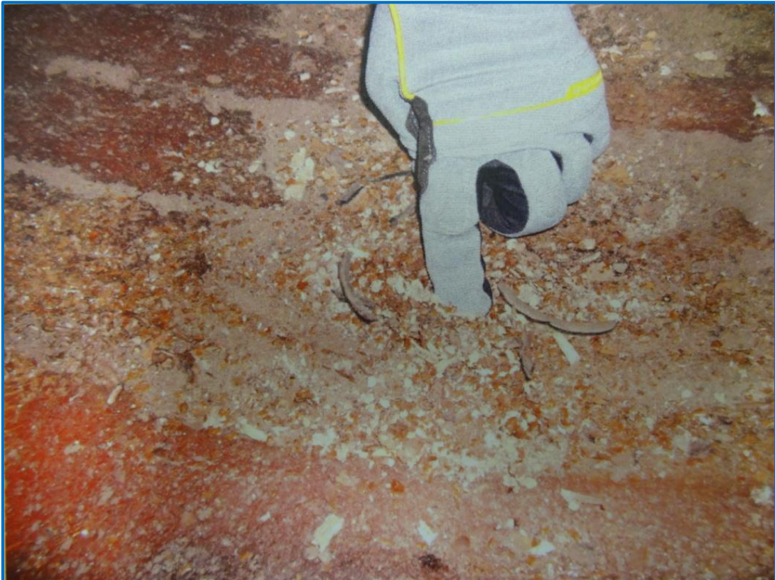
UST 87 Octane internal view: gel deterioration
