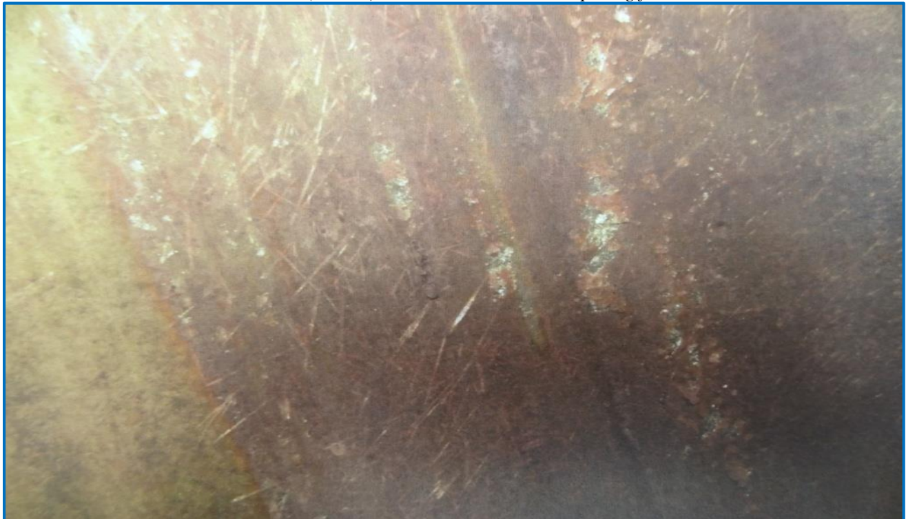
UST 87 Octane (master) - Gel-coat breakdown exposing fibers
