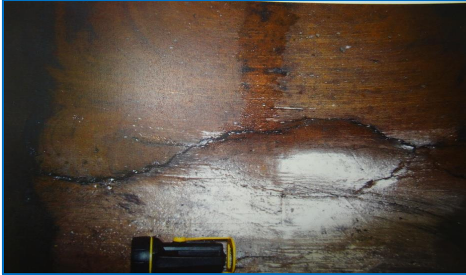
92 Octane UST interior – water entering tank through crack
