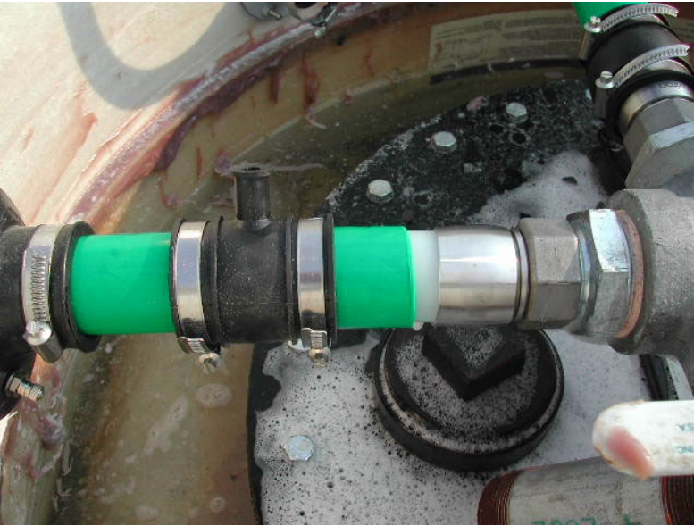
Double wall piping with test boots
