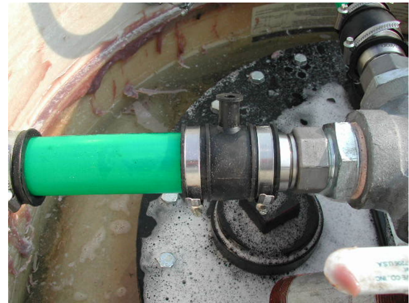
Double wall piping with test boots
