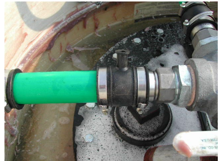
Double wall piping with test boots
