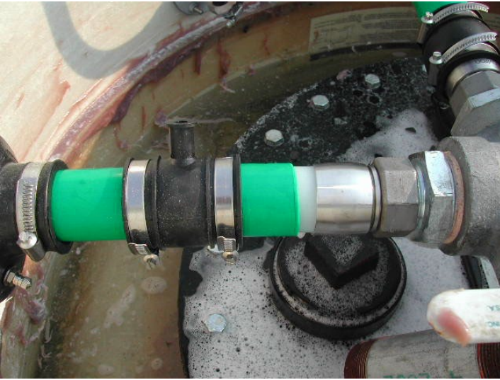
Double wall piping with test boots
