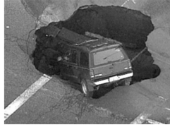
Sink hole caused by 8-in main break
