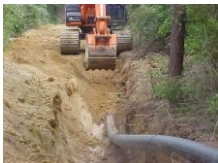
HDPE pipe installation
