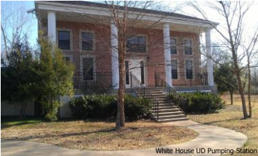
White House UD Pumping Station
