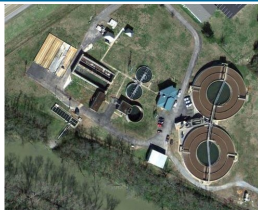
Fayetteville Wastewater Treatment Plant
