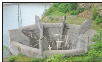
Watauga Dam Morning Glory spillway.
