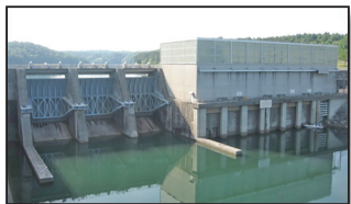
Melton Hill Dam and Powerhouse.
