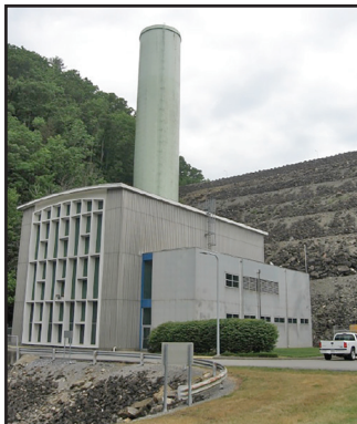
South Holston Dam, powerhouse, and surge tank.
