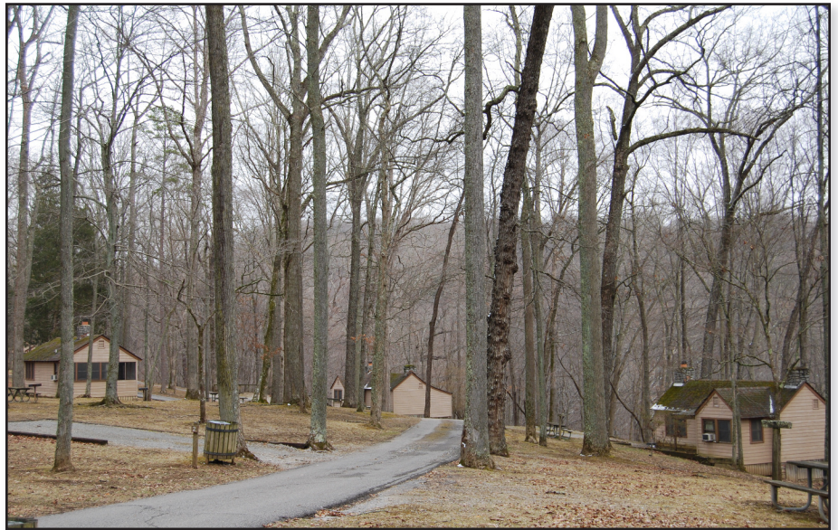
Norris Dam State Park Rustic Cabins Historic District, view to the east
