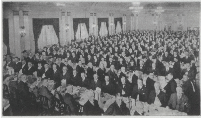
Banquet at the Hotel Fort Des Moines, January 11, 1921 Des Moines, Iowa
