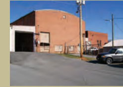
Figure 10. Shop at Langston School, Washington County. It is the only surviving shop we found and is now used as a county garage.
