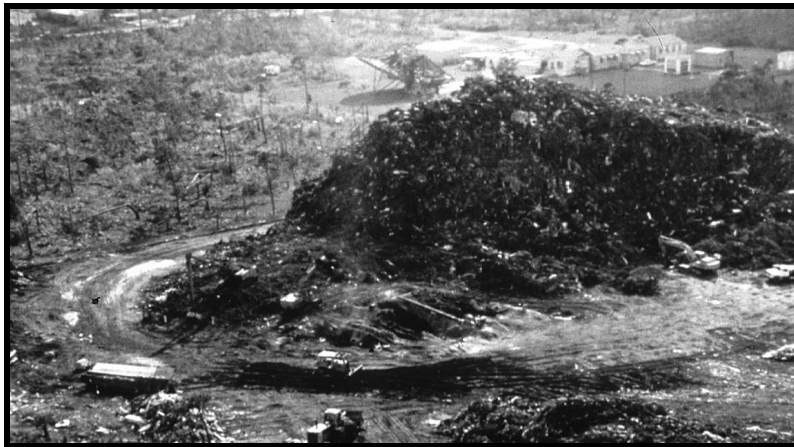
Figure 8.2 - DMS With Undesired Debris Accumulation
