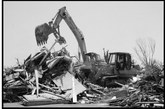
Figure 3.2 - Construction and Demolition Debris
