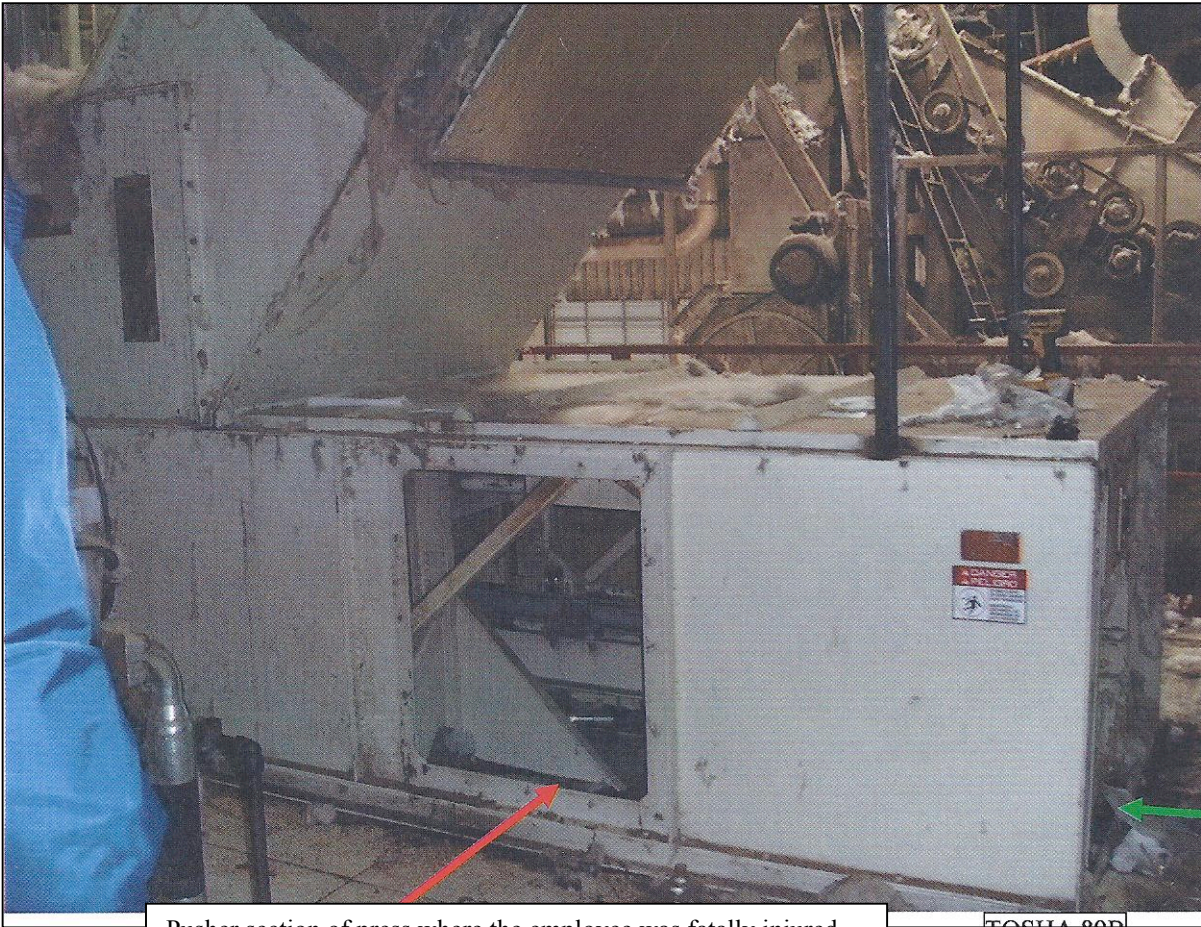
Pusher section of press where the employee was fatally injured.
