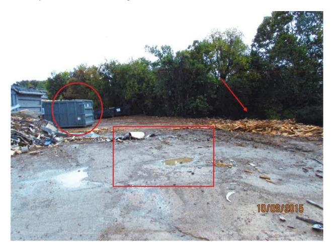
Photo 2 of 2 – This photo shows the area where the excavator was being operated (red square). The wood pile (red arrow) on the right was being loaded into a roll off dumpster (red circle) on the left. There was not type of barricading being used to keep employees clear of the boom's swing radius.
