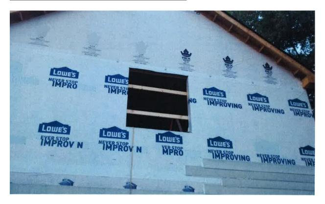
Photo 1 of 1 – The window opening just after the fall incident. Two 2x4's were in place at the time of the incident. Lower 2x4 measured 42 ½" from the floor and the upper 2x4 measure 69" from the floor of the detached garage.
