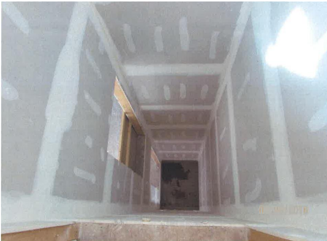
Photo 1 of 1 – Photo of the third floor elevator shaft
