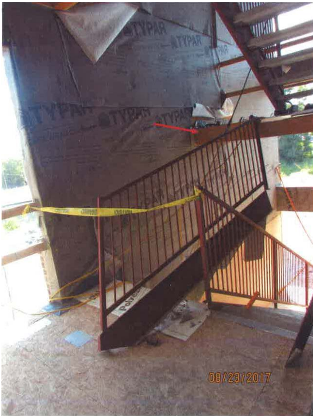
Photo 1 of 1 – Location of kick plate installation.
